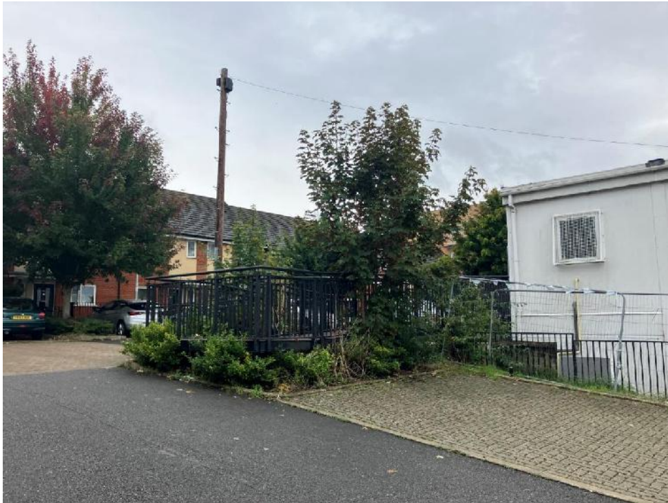
Photograph 1: Overview of T2
