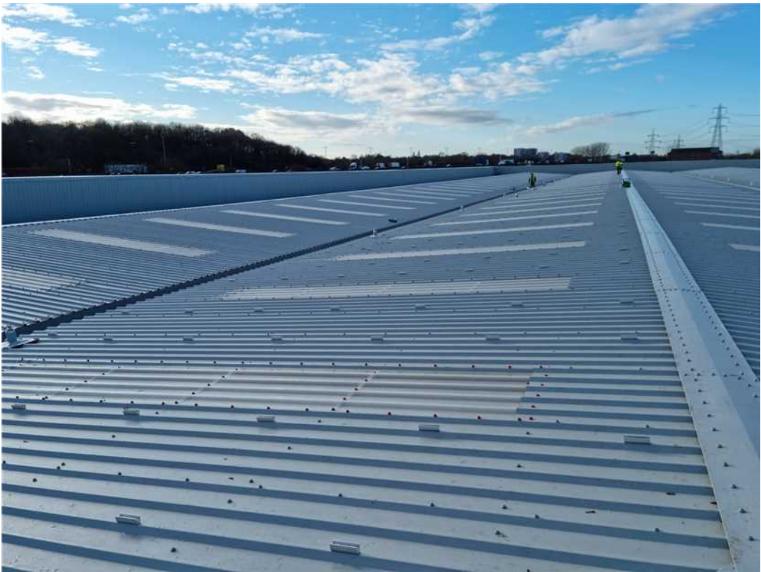
U-Supports fixed to crests of trapezoidal profile sheet
