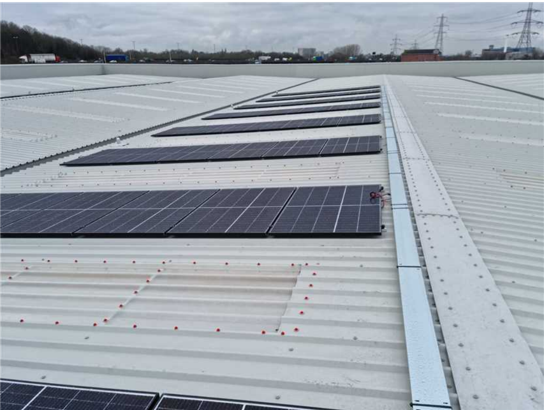
Panels clamped to U-supports
