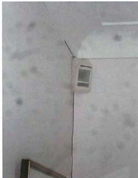
Cracking at extension junction in front reception.
