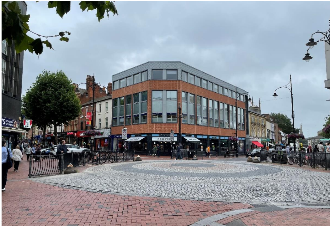
Figure 1.2: St Mary's House, Broad Street (the Site)
