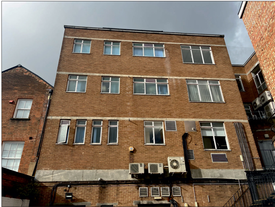
Photograph 2: Showing the rear of the building.
