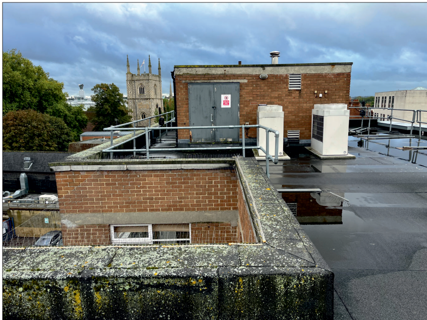
Photograph 3: Showing the flat roof and service unit.
