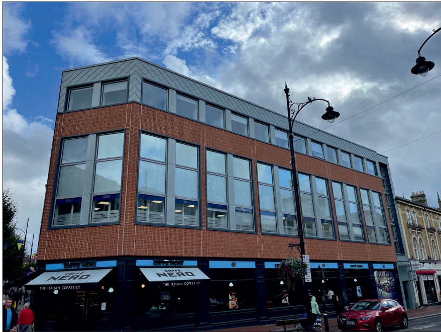
Photograph 1: Showing the front of the building.
