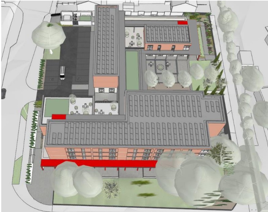
External 3D – canopies removed highlighted in red
