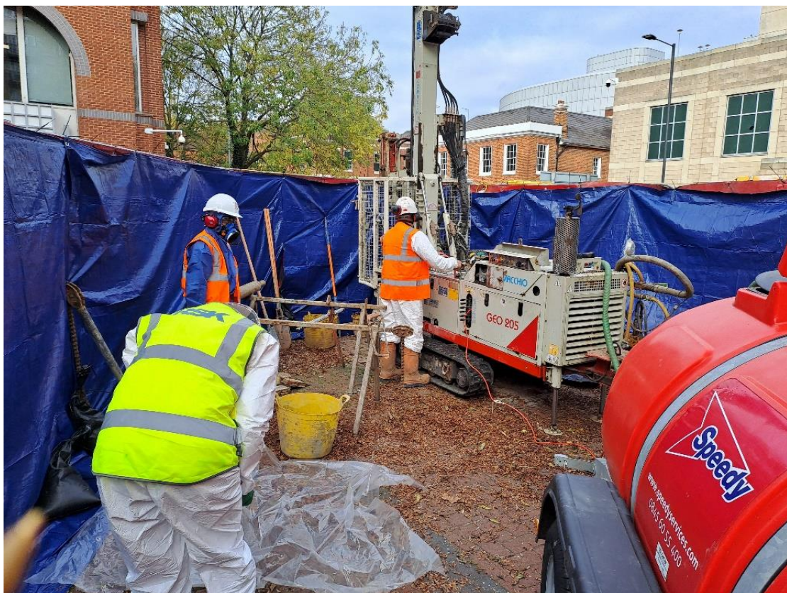
Figure 1: Working shot of BH203
