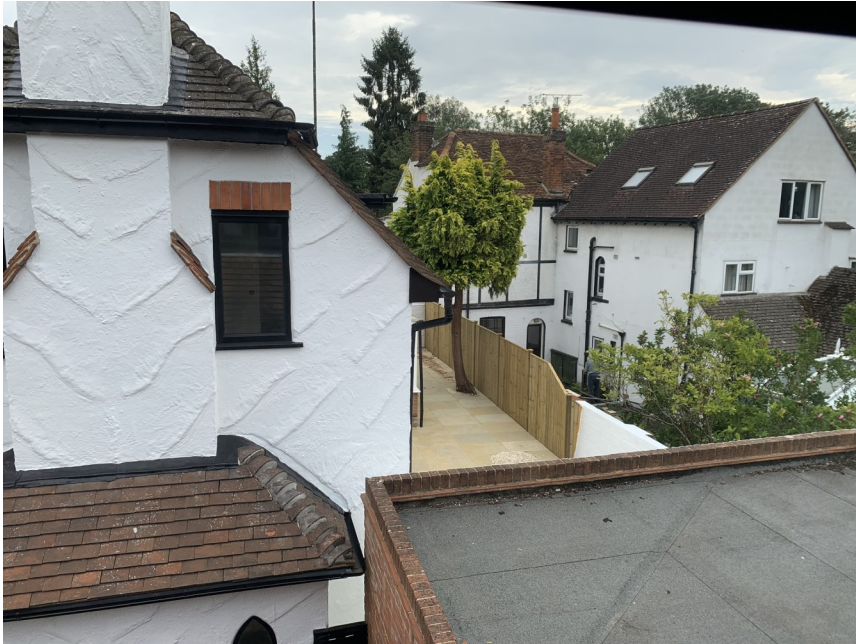
Overlooking of 18a garden from existing dormer to be removed
