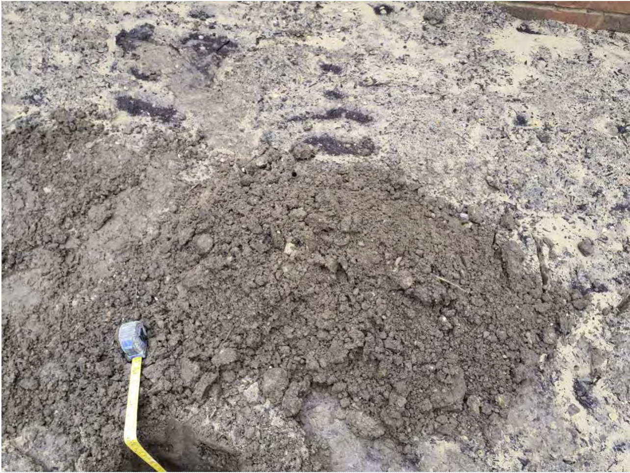
Photo of hole with tape in place
