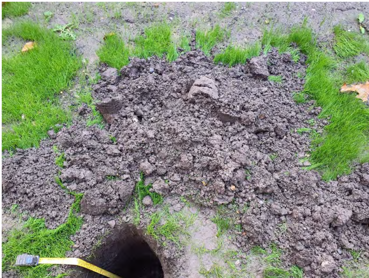
Photo of hole with tape in place
