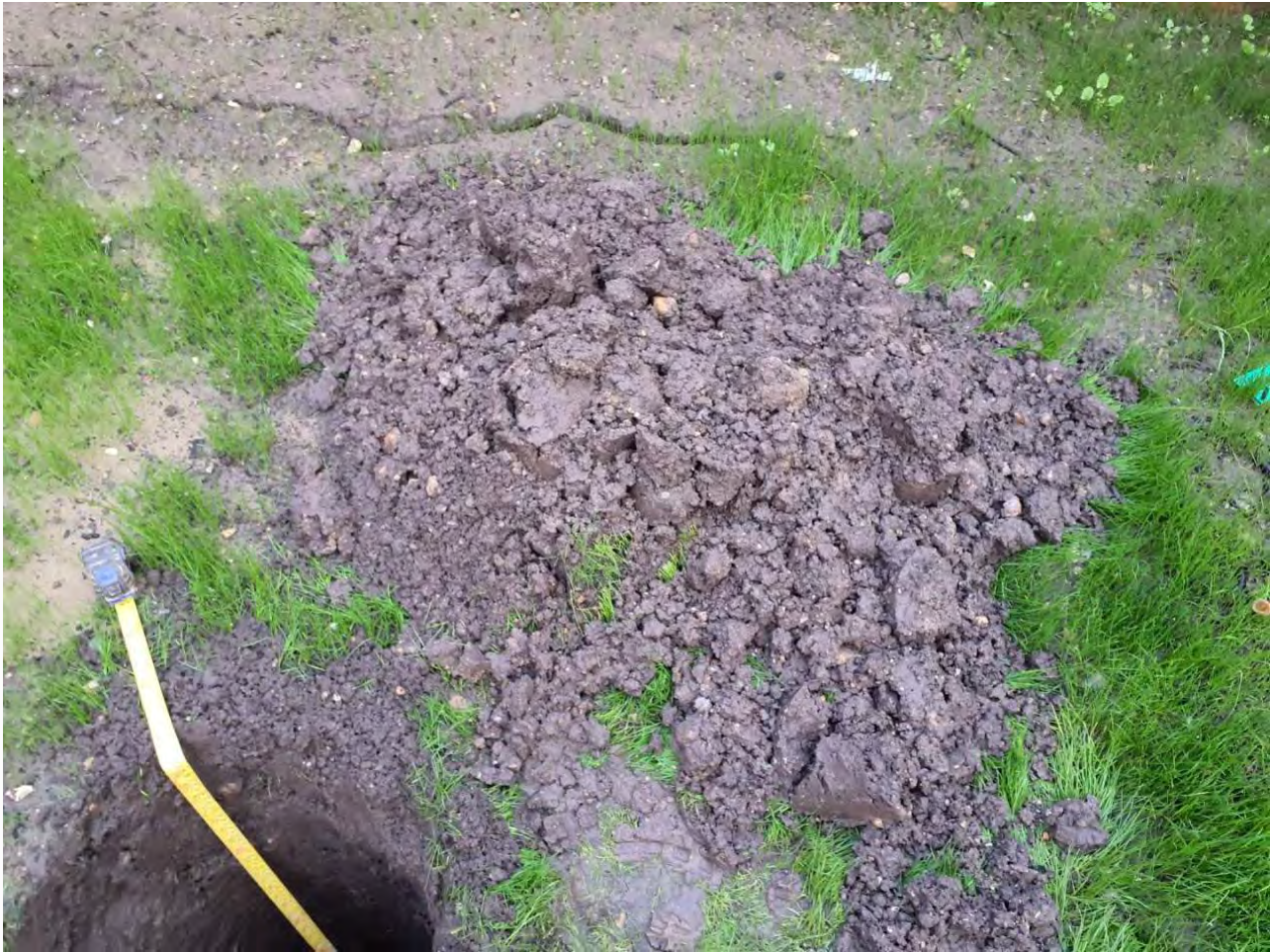
Photo of hole with tape in place
