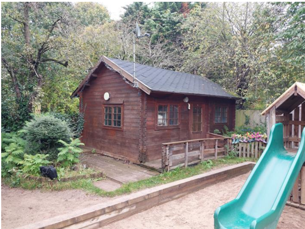
Photo 2: Existing outbuilding in north east corner
