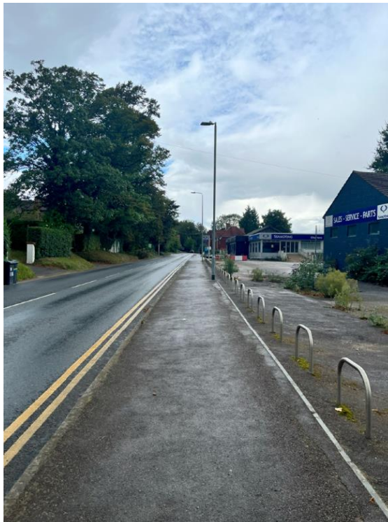
Image 3.2: Existing Footway Condition (Site Frontage)
