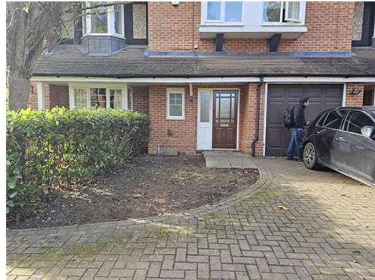
Existing garage frontage
