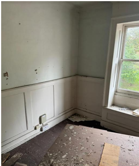
Fig. 48: View, looking north-west within the western second-floor room, with sash window and dado panelling.
