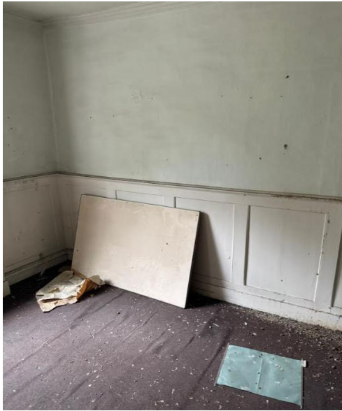
Fig. 47: View, looking north-east within the eastern second-floor room, with dado panelling and walls.
