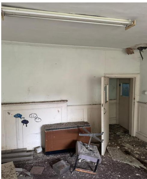
Fig. 49: View, looking south in the eastern second-floor room, with fireplace and doorway.
