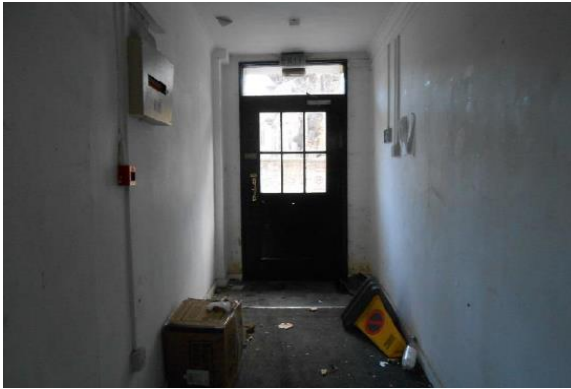
Fig. 8: View, looking north along the ground-floor central passageway, with the front door.
