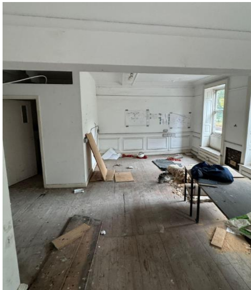
Fig. 38: View, looking west across east and west first-floor rooms, with inserted modern kitchen to the left.
