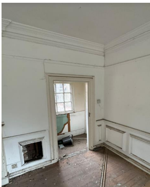
Fig. 39: View, looking south-west within the western room, with original doorway, dado and plaster cornice.
