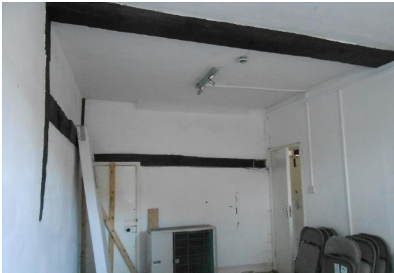
Fig. 9: View, looking south within the eastern ground-floor room, with exposed timber framing.
