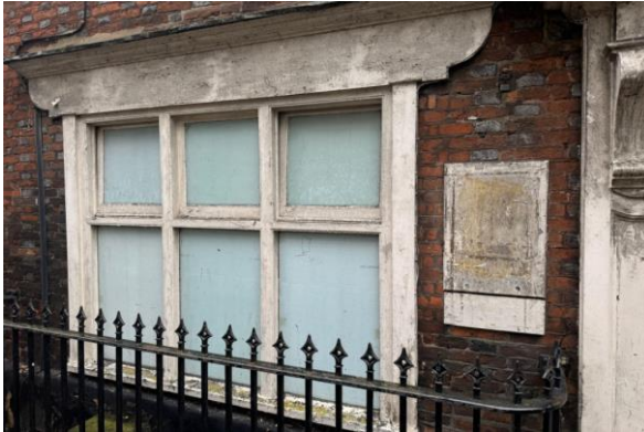
Fig. 12: Detail of the left-hand, timber-mullioned shopfront window.
