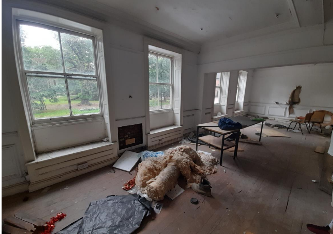
Fig. 36: View, looking north-east, of the first-floor interior of No. 10 Gun Street.
