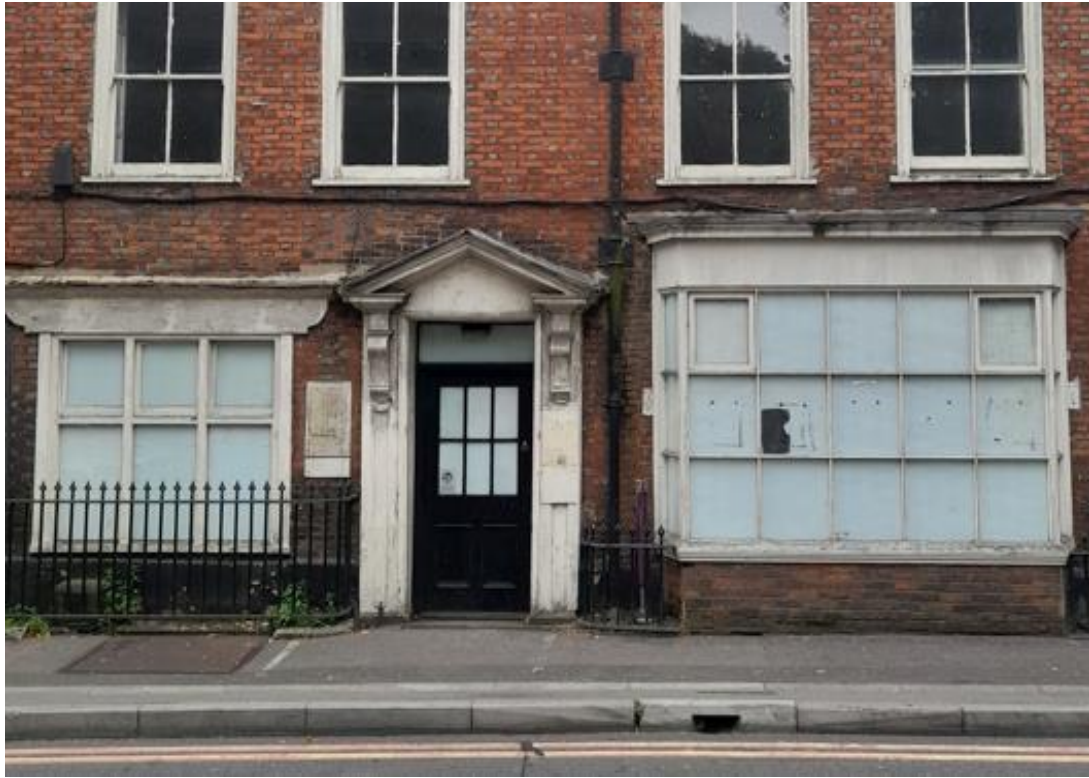
Fig. 4: The front doorway and two ground-floor shop windows of No. 10.
