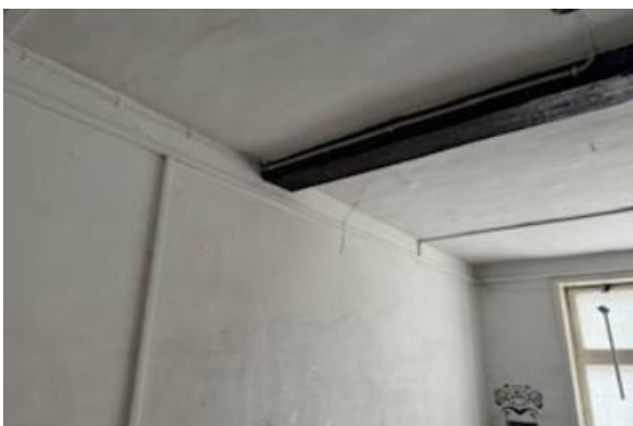
Fig. 11: View looking north-west within the eastern ground-floor room, with timber beam and moulded cornice.
