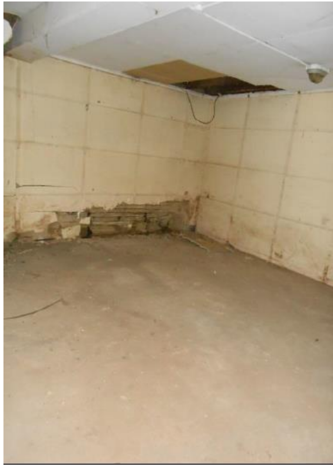
Fig. 6: View, looking north-east within the basement, with modern floor and surfaces.
