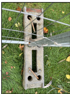
Protective Barrier (P.B.) Rubber feet will be used for the Heras fencing panels, which will be pinned into the ground using a soil pin. If the ground is impenetrable, the stabilisation bars will be mounted on a block tray and suitably weighted.
