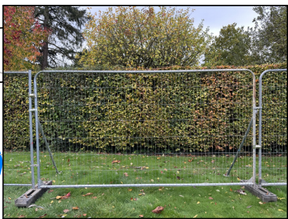
Protective Barrier (P.B.) Heras fencing panels.
