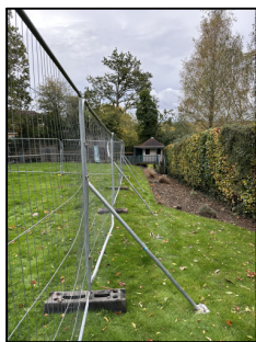
Protective Barrier (P.B.) A support bar will be placed at a 45-degree angle at each end of the Heras panel and pinned to the ground using a soil pin.
