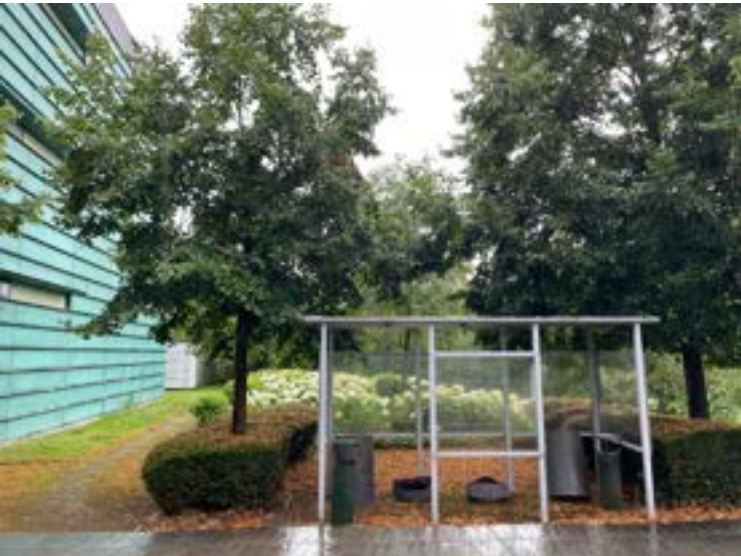
The existing smoking shelter to the north of the building
