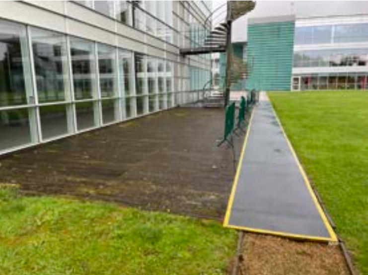
Communal decking along the western side of the building
