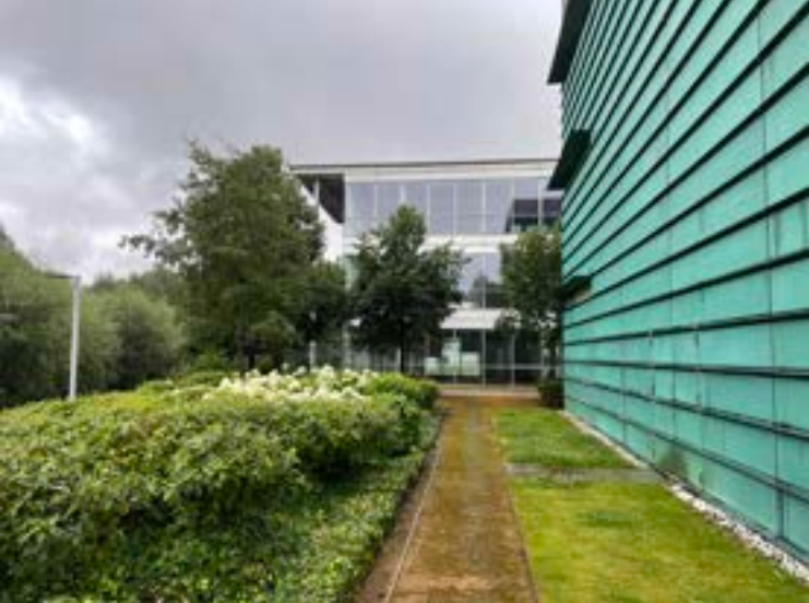
The path along northern facade to the rear courtyard
