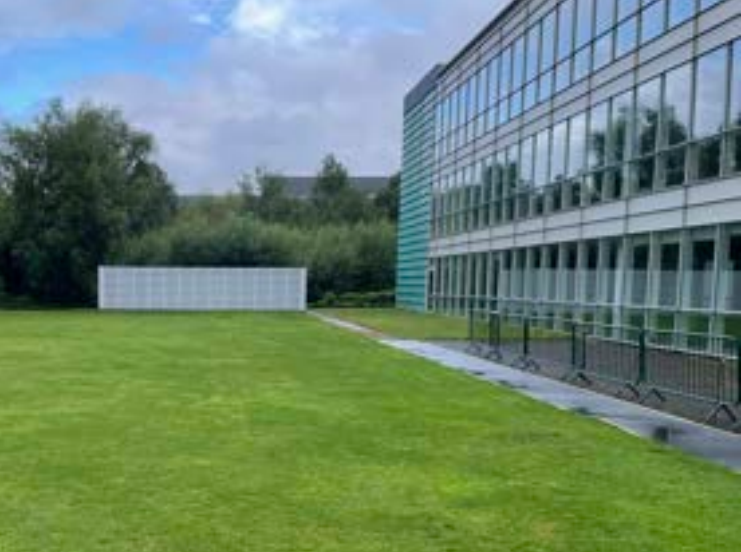
Fenced off plant area on concrete base to be removed.
