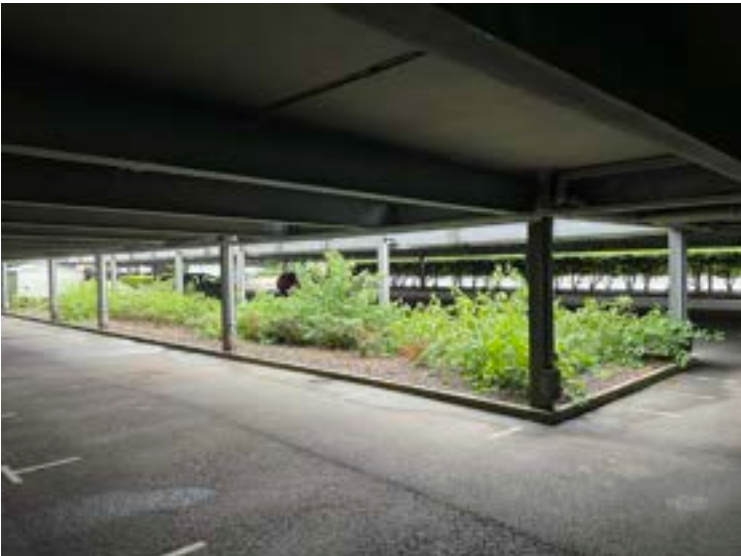
The light well in the middle of the car park
