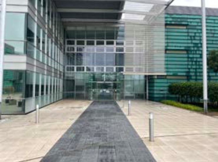
The main entrance of 300 Brook Drive
