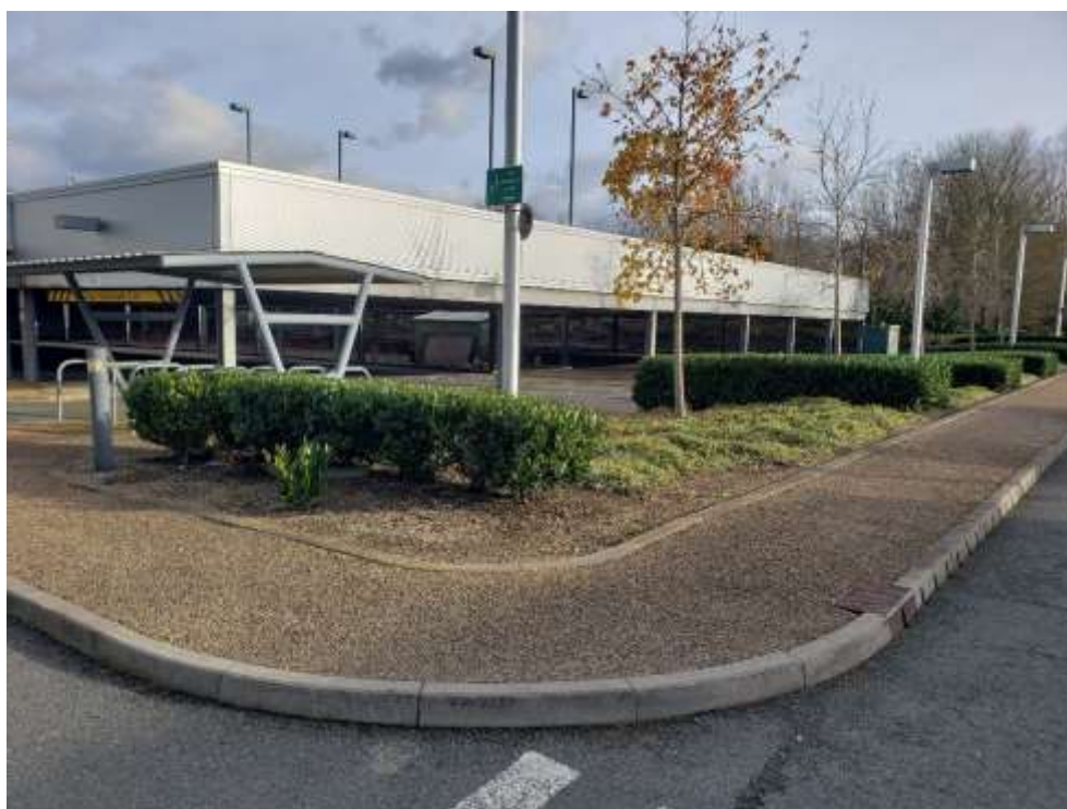
Photograph 2 - Two storey car park
