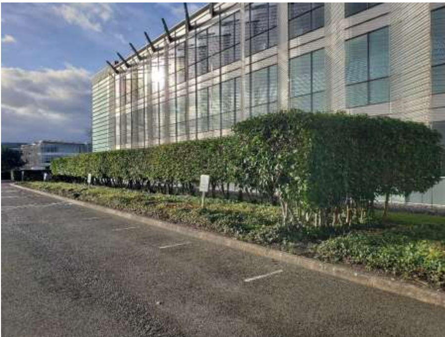
Photograph 1 - Building with shrubs and hardstanding in the foreground
