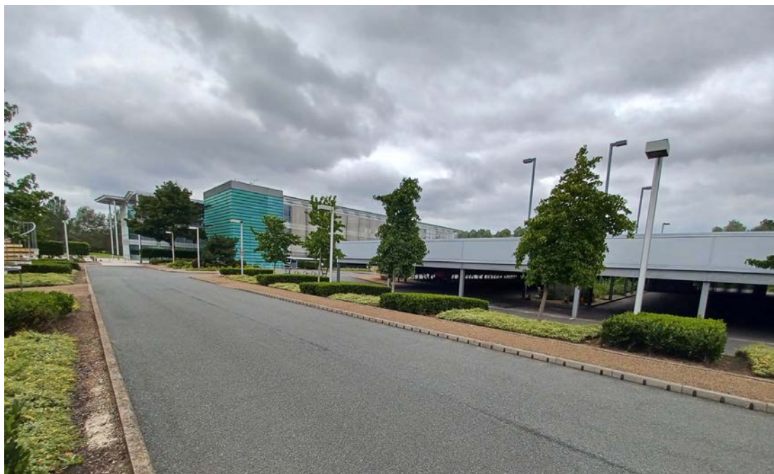
Main approach showing Multi-storey car park.
