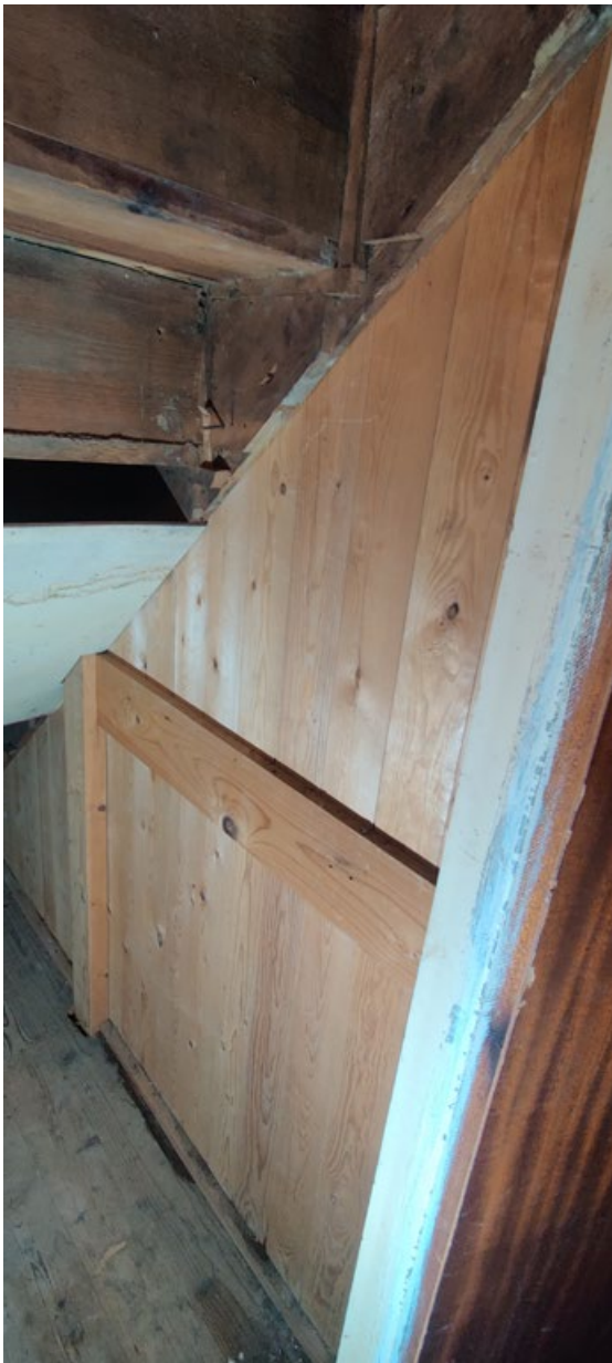
Evidently new support structure cladding for staircase
