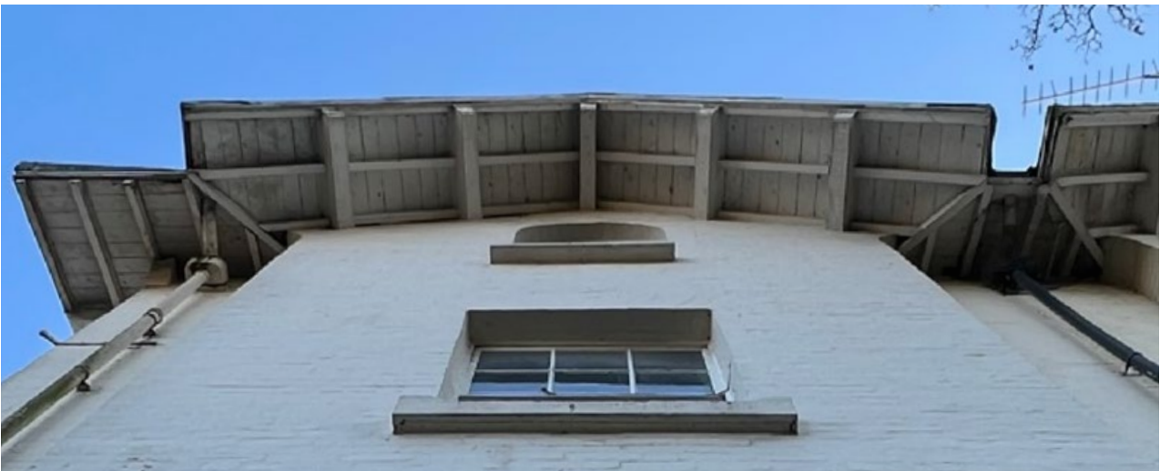
Eaves also typical of the Eldon Square Conservation Area
