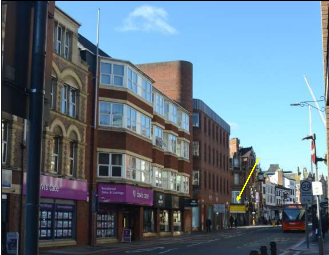
Figure 23: View of 2-4 Kings Road looking west along Kings Road into the conservation area (ground floor of site highlighted in yellow)
