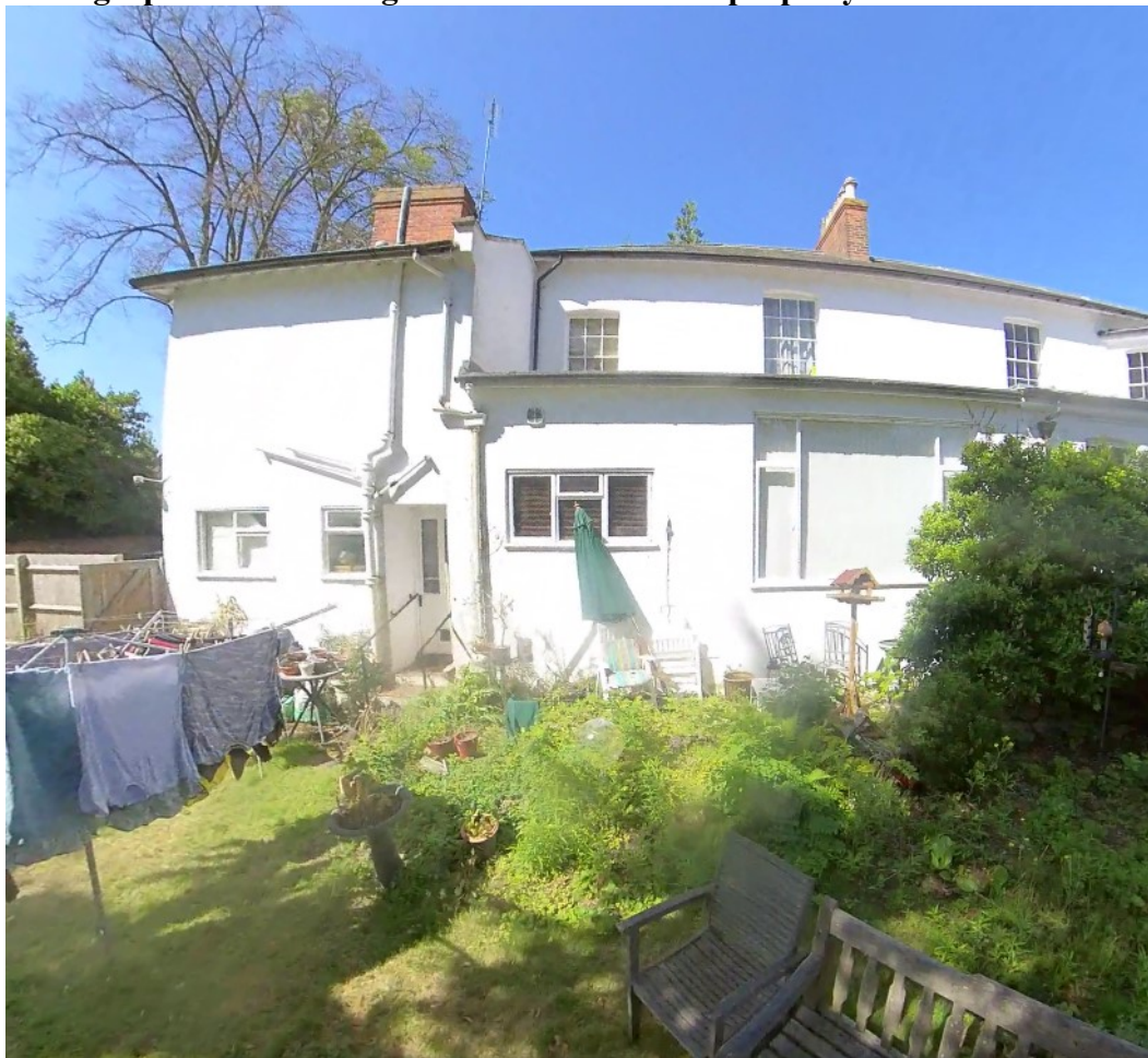
Photograph of the existing rear elevation of the property
