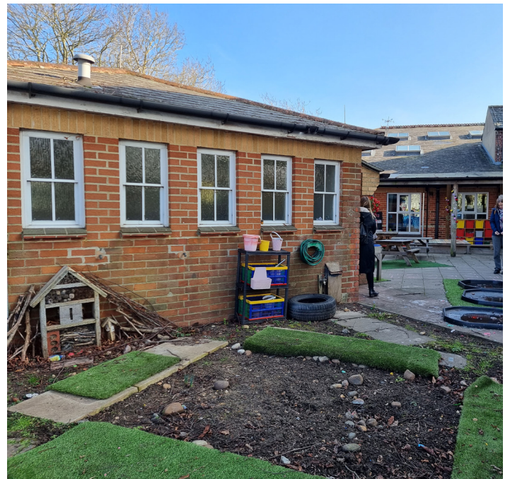
Fig. 04 - Yr 1 classroom/toilet - 1930's/1950's extension
