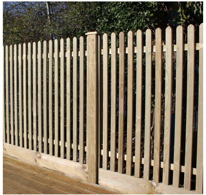
Fig. 09 - Example of 1.2m timber palisade fencing
