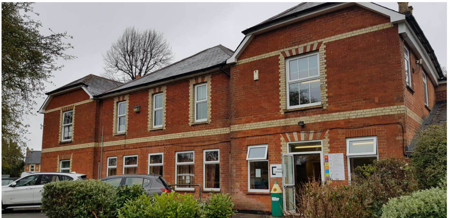
Fig. 02 - Main two-storey block, originally 'The Laurels'. Pre-1870's, South elevation
