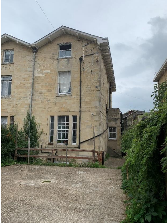
Rear Elevation of 6 Eldon Road
