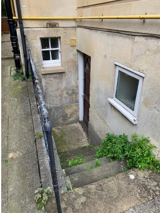
View of entrance to the basement flat
