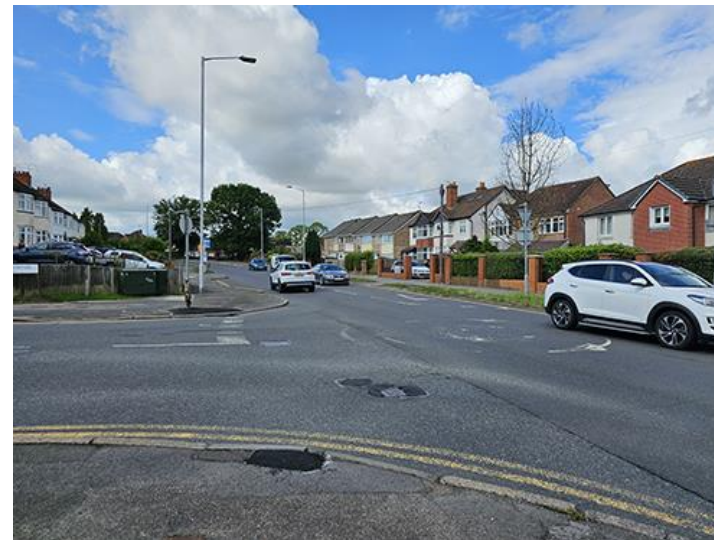
Highway view south
