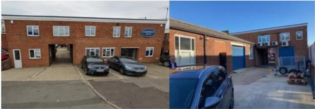
1.10 The existing front and rear of the site.
