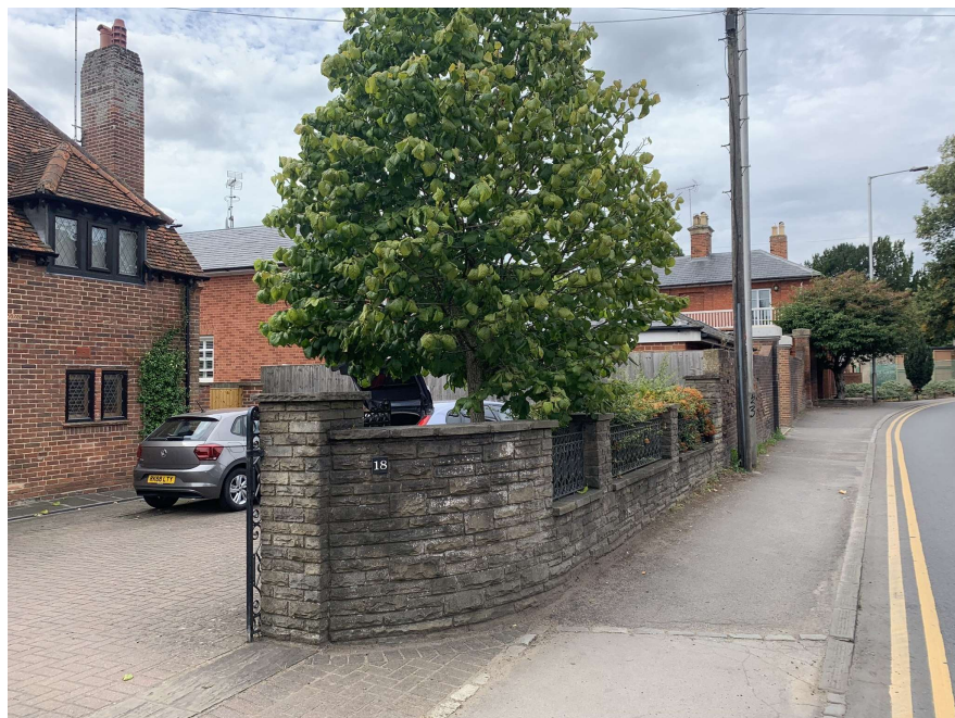
Existing Boundary Wall To no. 18 (non original)
