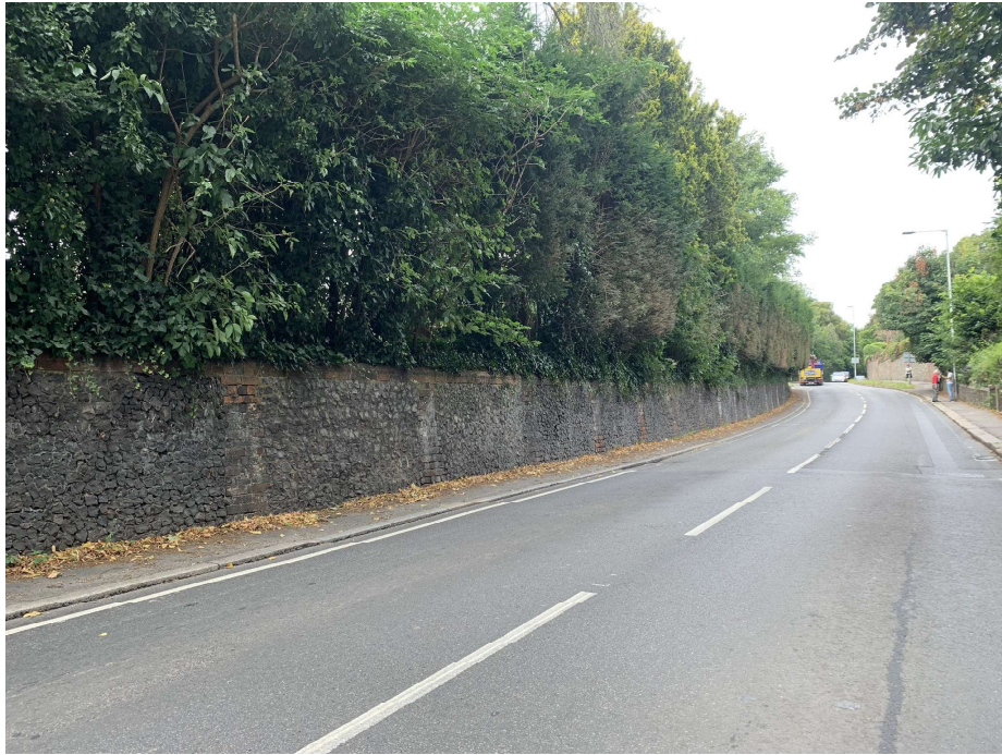
St Peters Hill Flint Boundary Wall
