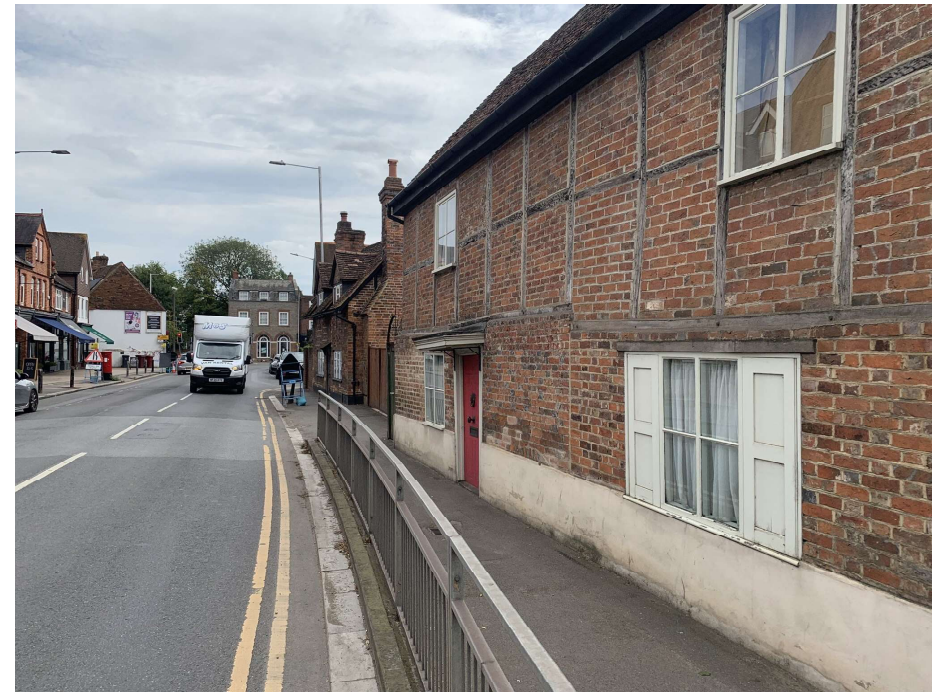
Neighbouring Properties Red Brick Wall Abutting Highway
