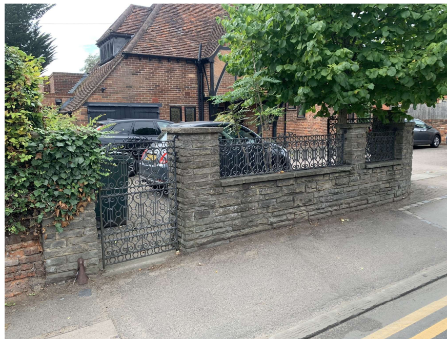
Existing Boundary Wall To no. 18 (non original)
