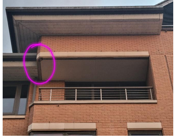
Figure 3: Roof of balcony on northern aspect
