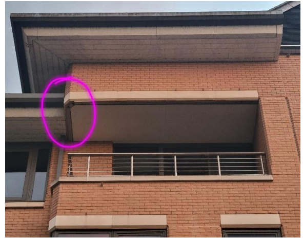
Figure 16: Roof of balcony on northern aspect
