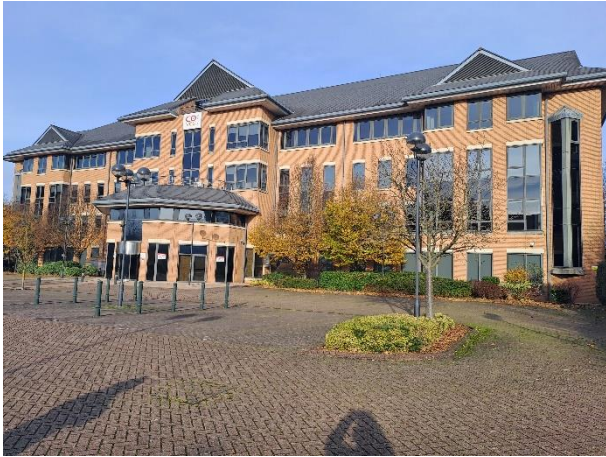
Figure 10: Building B1 – Southern aspect
