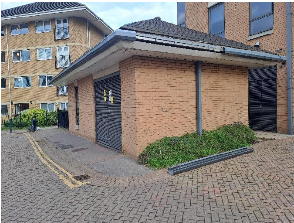
Figure 14: Building B3 – Southern and western aspects
