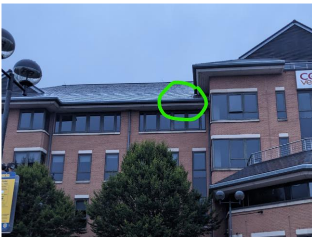
Figure 4: Roof tiles on southern aspect
