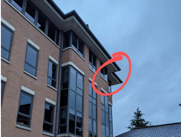
Figure 2: Soffit on south-east corner
