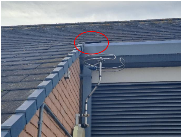
Figure 11: Building B1 – A lifted roof tile on the northern aspect
