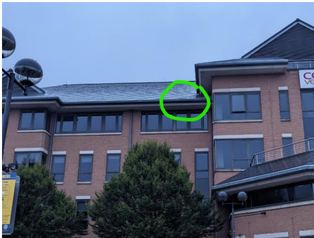
Figure 17: Roof tiles on southern aspect
