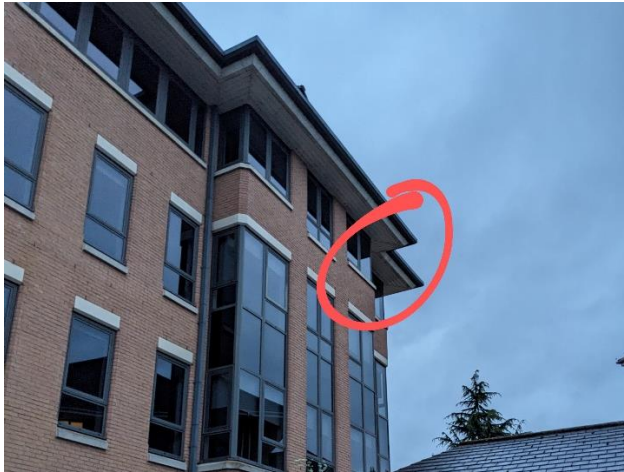
Figure 15: Soffit on south-east corner
