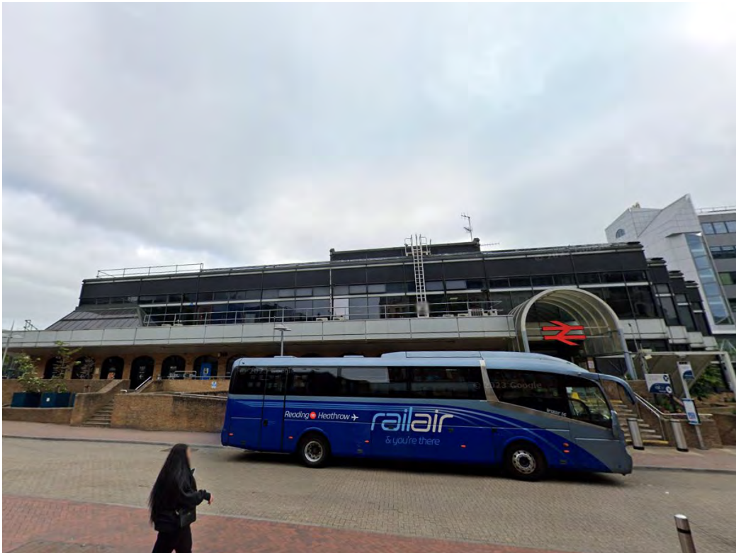
3 Entrance to Waiting Lounges and RailAir Services
