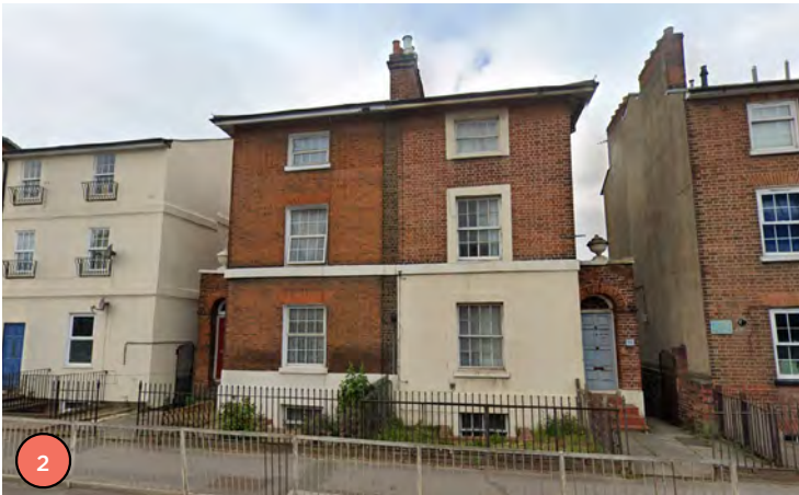
29 & 31 Caversham Road, 1847 (Grade II)
