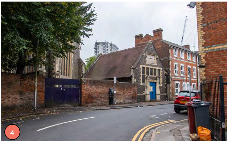
Quadrant Walls & Railings to former No.64 (Greyfriars Vicarage), 1796 or 1808 (Grade II)
