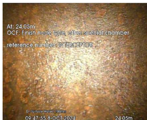
SW1 DOWNSTREAM INTERCEPTOR_24-05m_094755.jpg, 00:05:01, 24.05 m Finish node, other special chamber, reference: INTERCEPTOR, .
