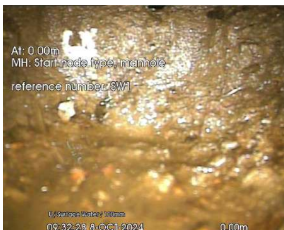
SW1 UPSTREAM LINE A_0-00m_093228.jpg, 00:00:05, 0.00 m
