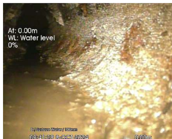
SW1 DOWNSTREAM INTERCEPTOR_0-00m_094129.jpg, 00:00:12, 0.00 m Water level, 0% of the vertical dimension
