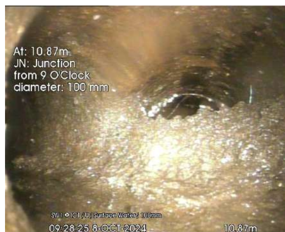
SW1 UPSTREAM IC1_10-87m_092825.jpg, 00:03:07, 10.87 m Junction at 9 o'clock, 100mm dia
