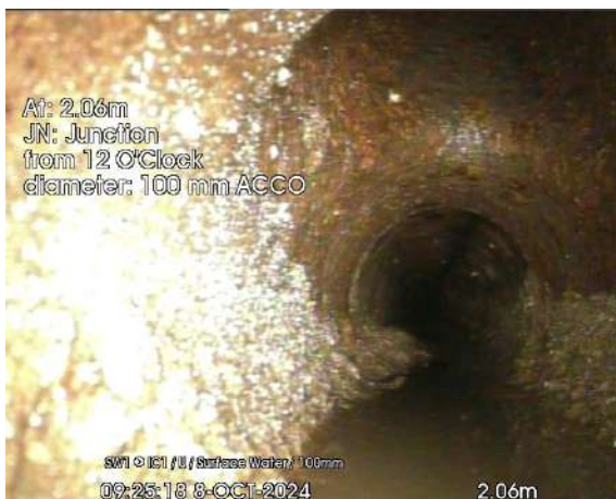
SW1 UPSTREAM IC1_2-06m_092518.jpg, 00:00:44, 2.06 m Junction at 12 o'clock, 100mm dia, ACCO
