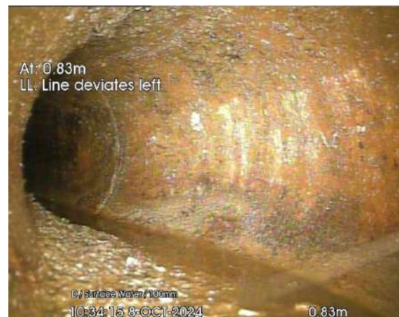
SW2 DOWNSTREAM INTERCEPTOR_0-83m_103415.jpg,
