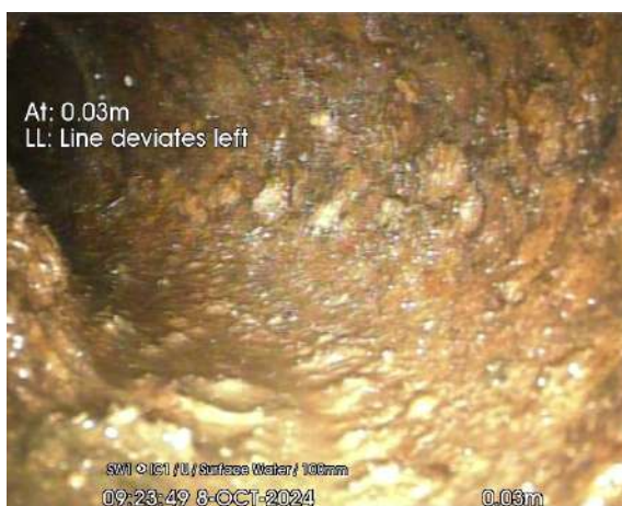
SW1 UPSTREAM IC1_0-03m_092349.jpg, 00:00:12, 0.03 m Line deviates left
