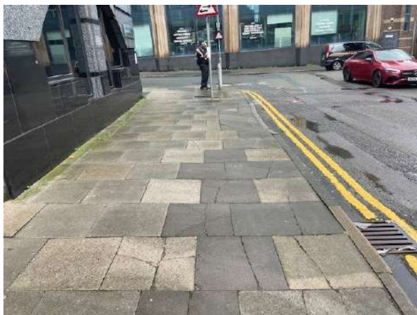
AREA OF PUMP AND FW LINE TO MAINS
