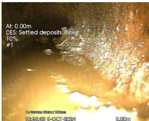
SW2 DOWNSTREAM INTERCEPTOR_0-00m_103353.jpg,
