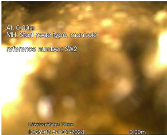
SW2 UPSTREAM LINE A_0-00m_102902.jpg, 00:00:05, 0.00m
