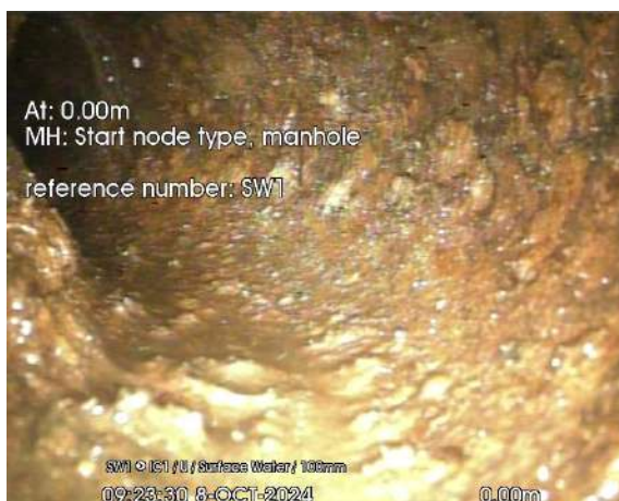
SW1 UPSTREAM IC1_0-00m_092330.jpg, 00:00:05, 0.00 m Start node, manhole, reference: SW1
