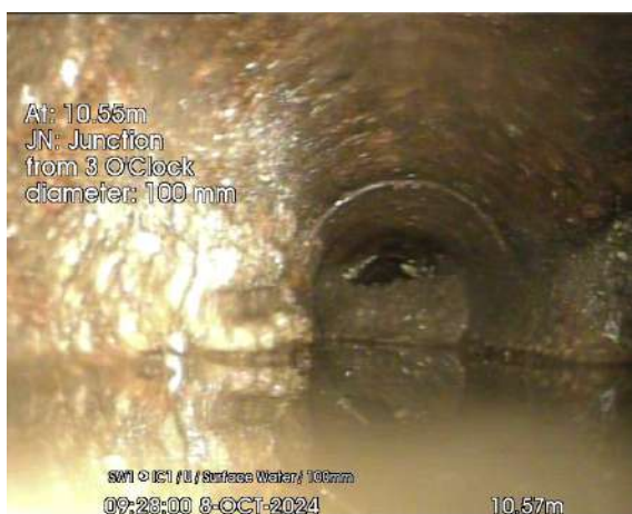
SW1 UPSTREAM IC1_10-57m_092800.jpg, 00:02:54, 10.57 m Junction at 3 o'clock, 100mm dia
