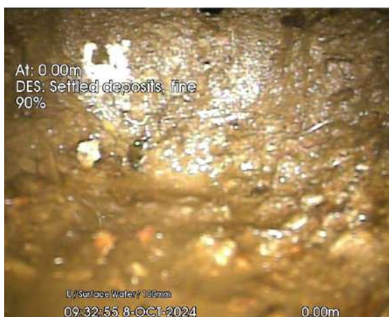
SW1 UPSTREAM LINE A_0-00m_093255.jpg, 00:00:14, 0.00 m
