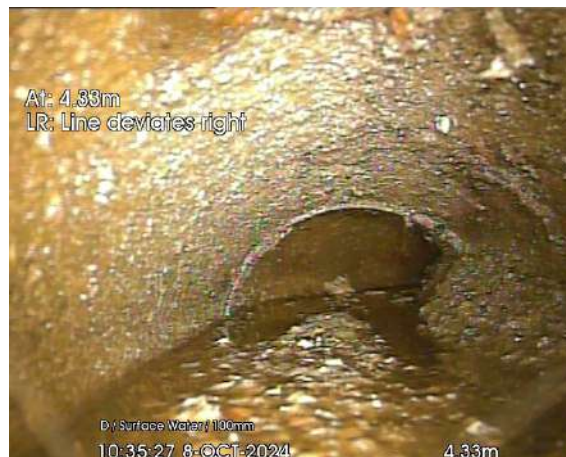
SW2 DOWNSTREAM INTERCEPTOR_4-33m_103527.jpg, 00:01:26, 4.33 m Line deviates right
