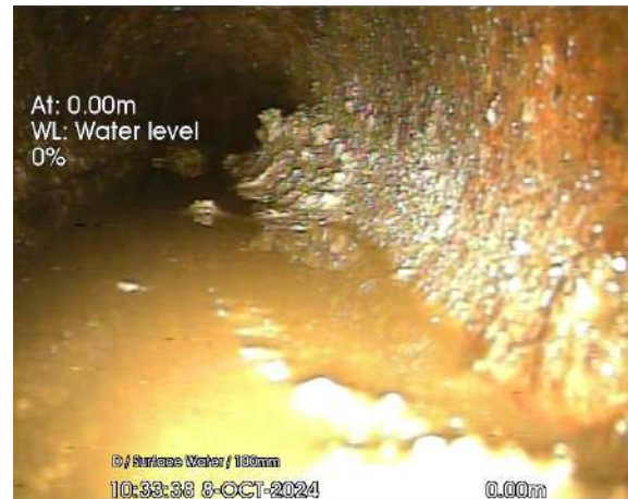
SW2 DOWNSTREAM INTERCEPTOR_0-00m_103338.jpg,
