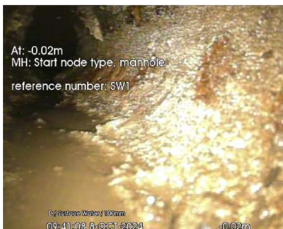
SW1 DOWNSTREAM INTERCEPTOR_-0-02m_094108.jpg, 00:00:04, -0.02 m Start node, manhole, reference: SW1
