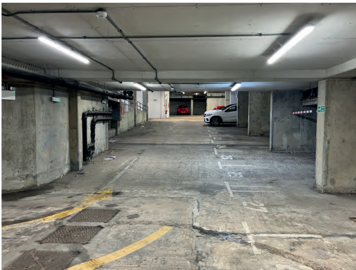
Plate 8: View from the north-western part of the study site in the below-ground carpark looking south
