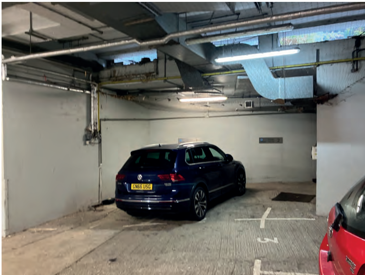
Plate 7: View from the south-western part of the study site in the below-ground carpark looking east
