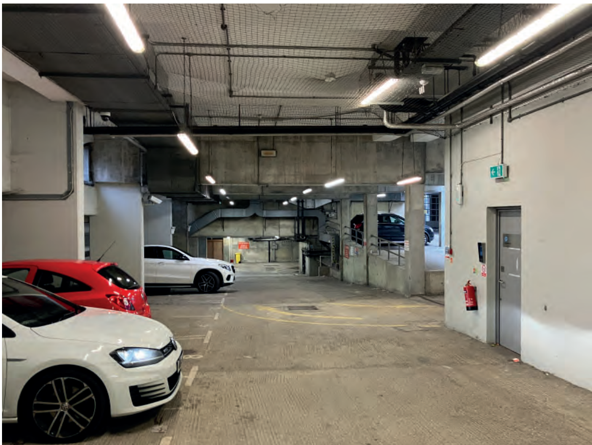
Plate 6: View from the south-western part of the study site in the below-ground carpark looking north
