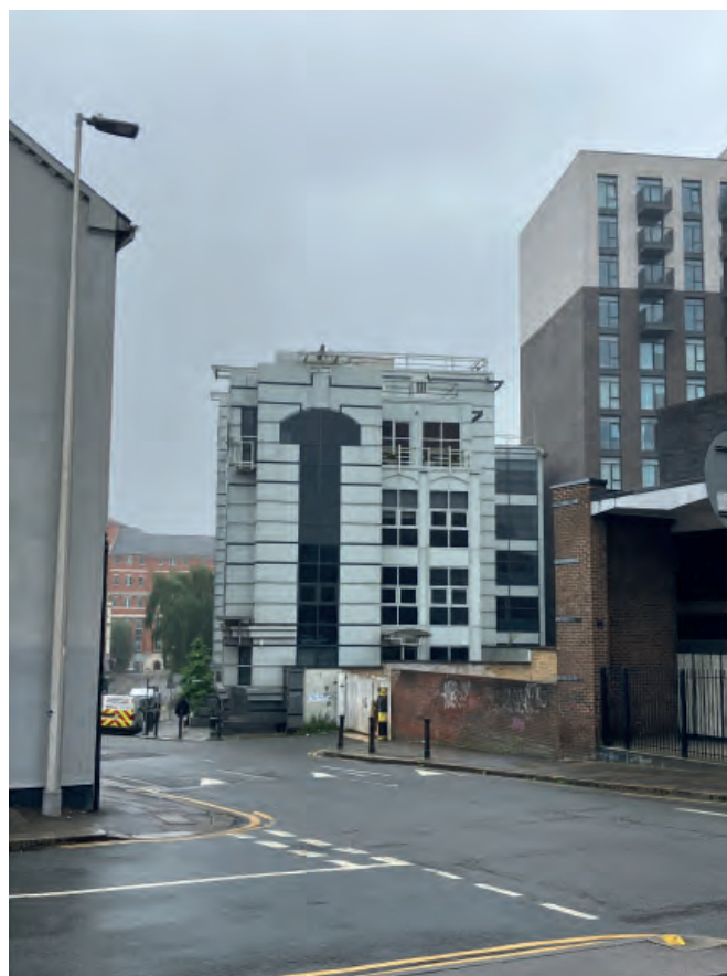
Plate 2: View from the junction of Sackville Street and Greyfriars Road looking north-east towards the study site
