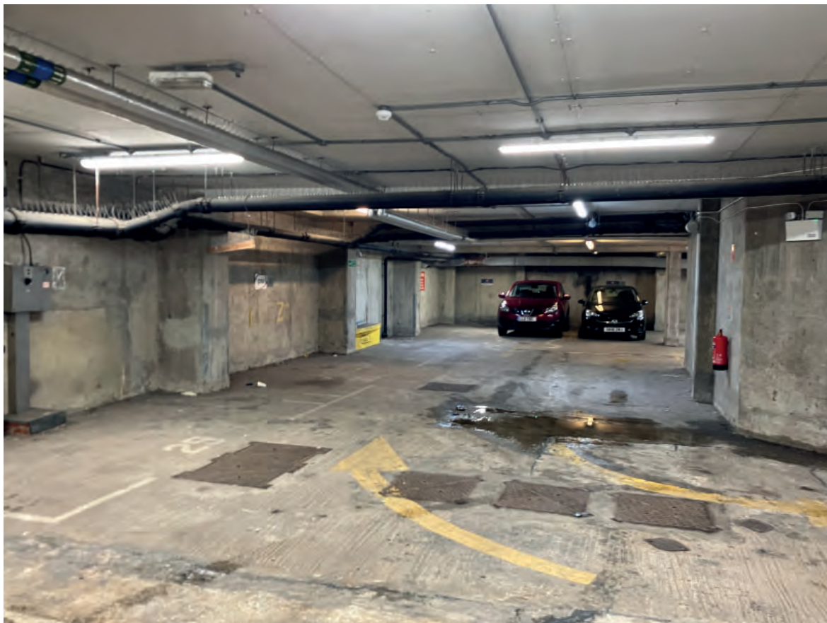
Plate 9: View from the north-western part of the study site in the below-ground carpark looking east
