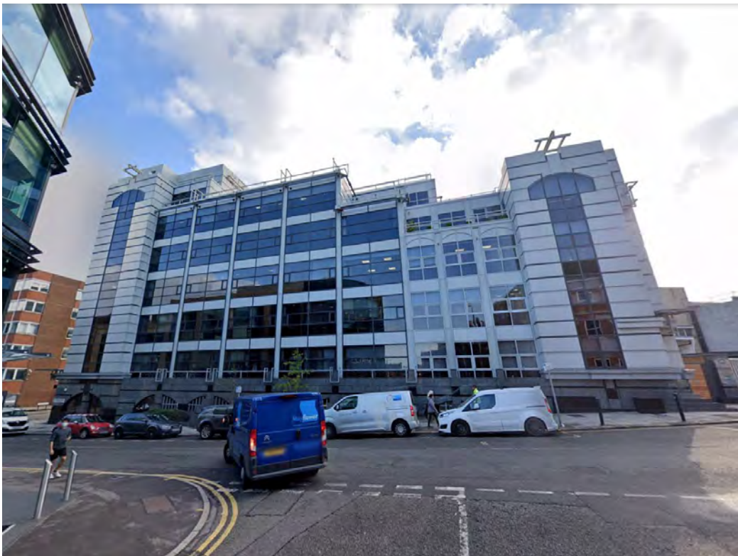
V3 The existing buildings west elevation.
