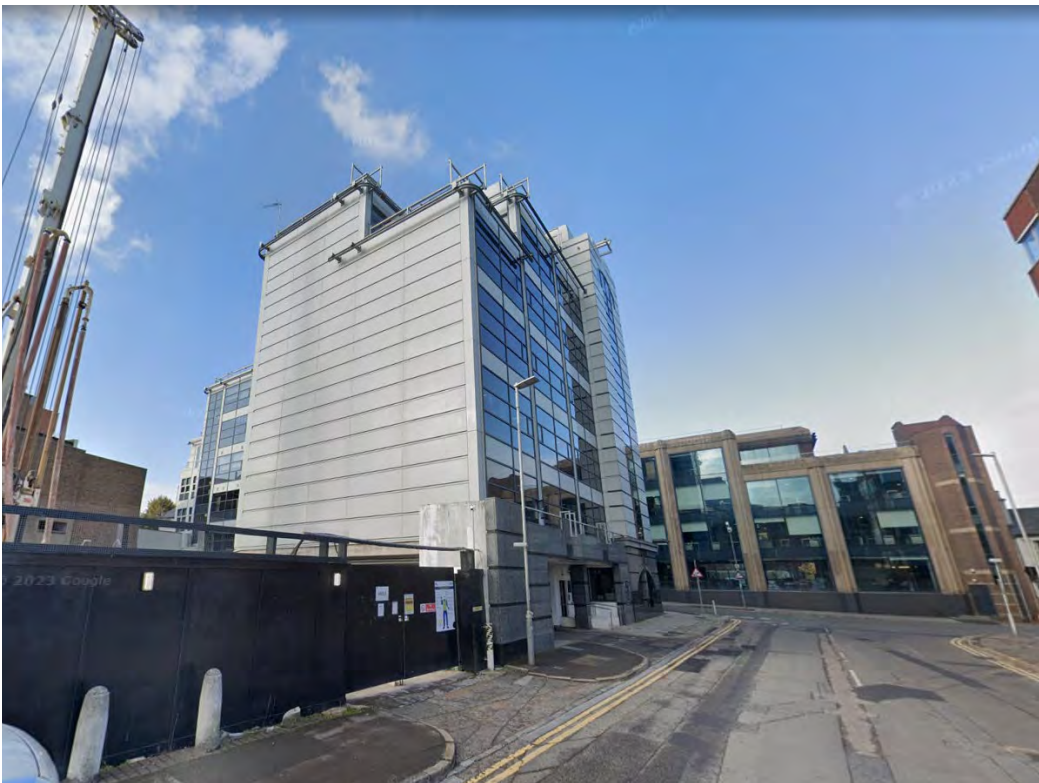
V4 The existing scheme's east elevation (prior to construction of Station Hill Development).
