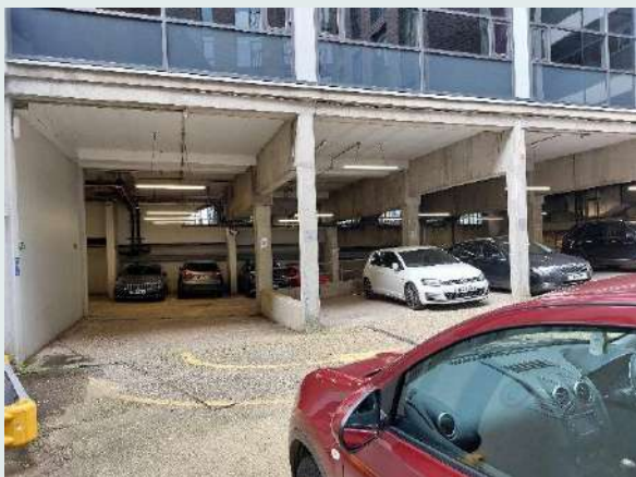
The Undercroft Car Parking towards the West
