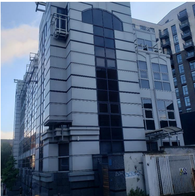
Figure 4.1 Building viewed from southern end
