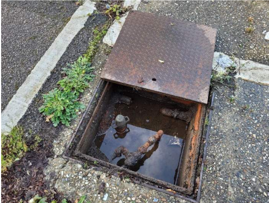
Photo 3 – Exposed tank entry (ref U7)
