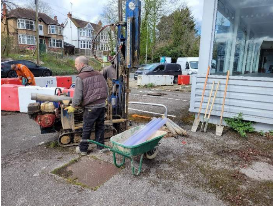
Photo 5 – Window sampling at location BH5
