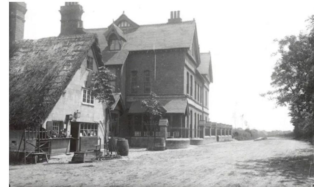
Fig. 1 The Roebuck Hotel, Oxford Road
