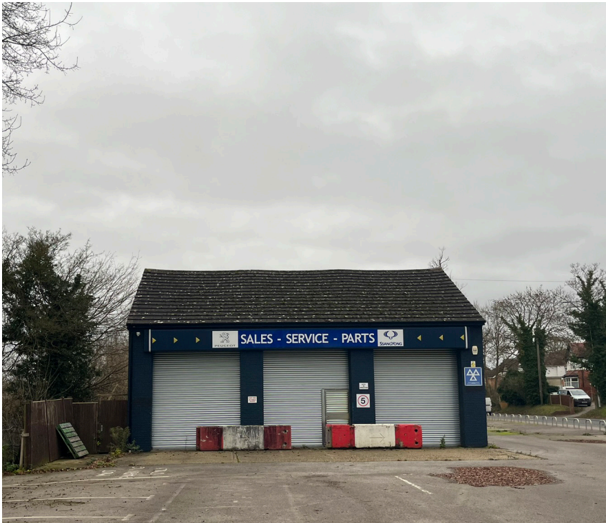
Open space for car servicing purposes
