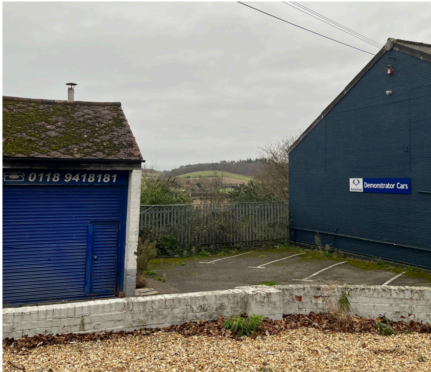
Blockwork separation between the site and Oxford road
