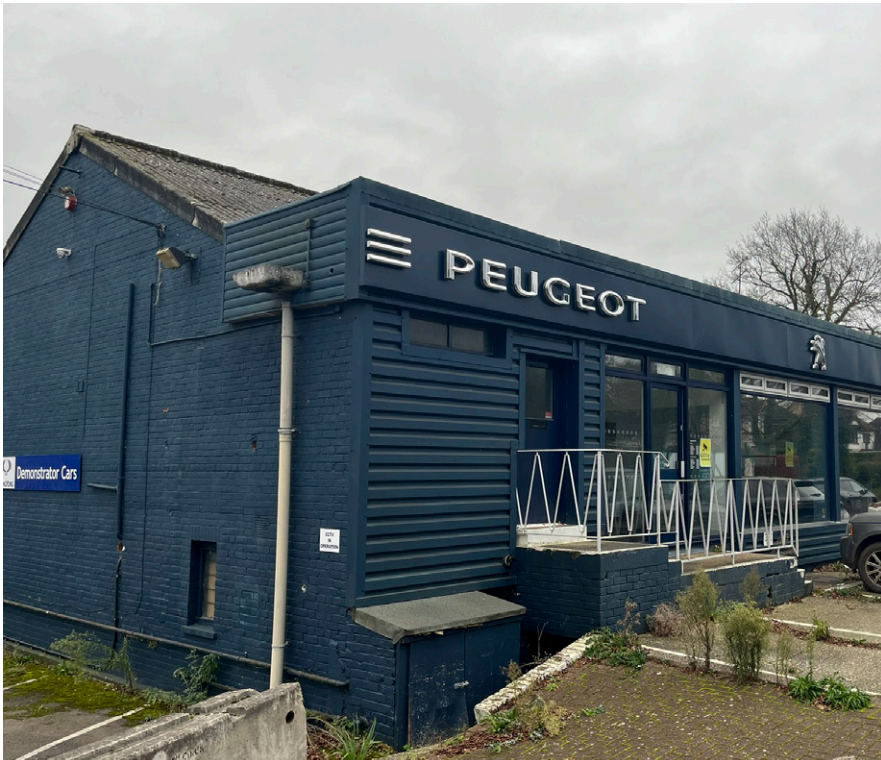
Existing building used for car dealership. Brickwork painted over. Flat roof annex to the original building
