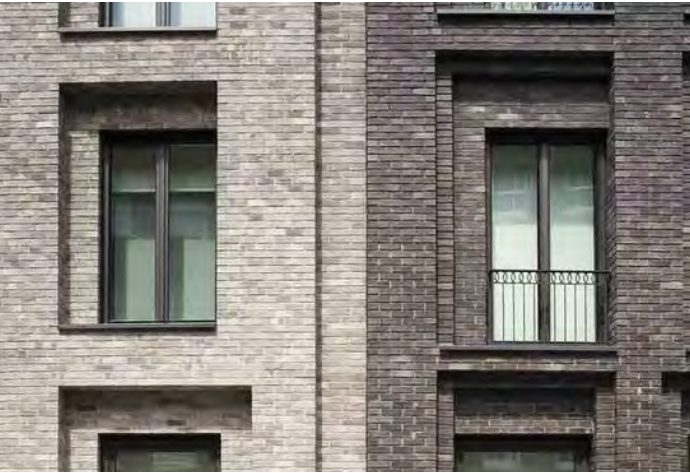
Ground Floor Active Frontage
