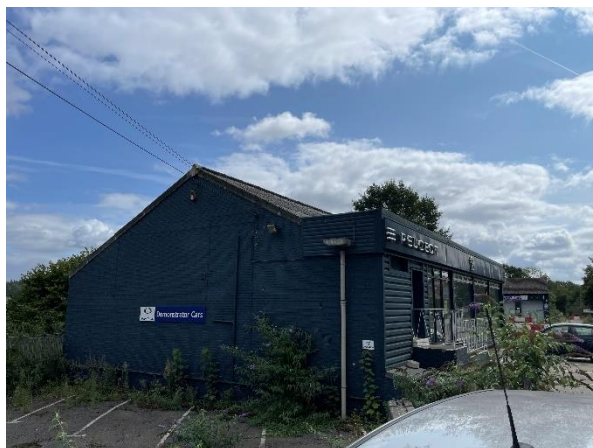
Photograph 4. Building 2 viewed from the south-west.
