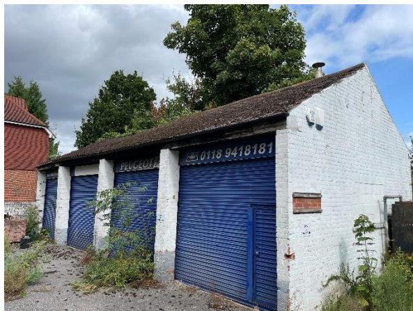
Photograph 2. Building 1 viewed from the south-east.
