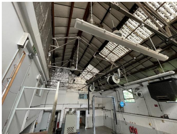
Photograph 8. The northern interior section of Building 2.
