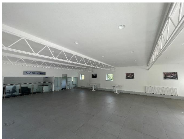
Photograph 6. The southern interior section of Building 2.
