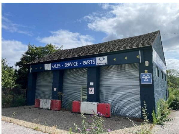
Photograph 9. Building 3 viewed from the south-west.
