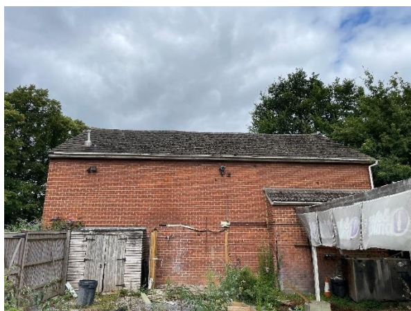
Photograph 10. Building 3 viewed from the east.
