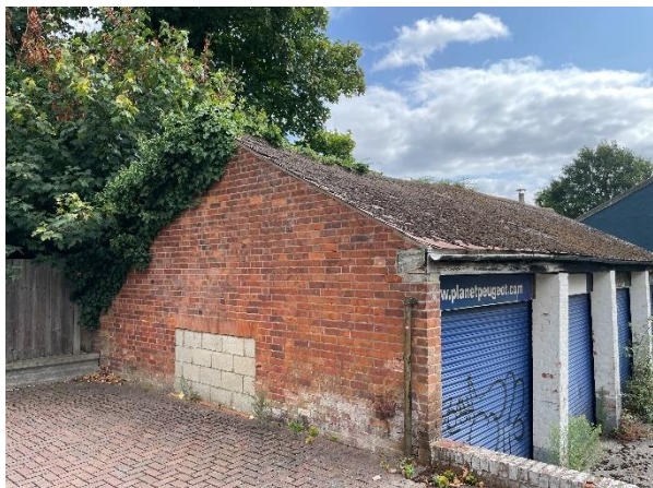
Photograph 1. Building 1 viewed from the south-west.
