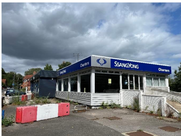
Photograph 5. Building 2 viewed from the south-east.
