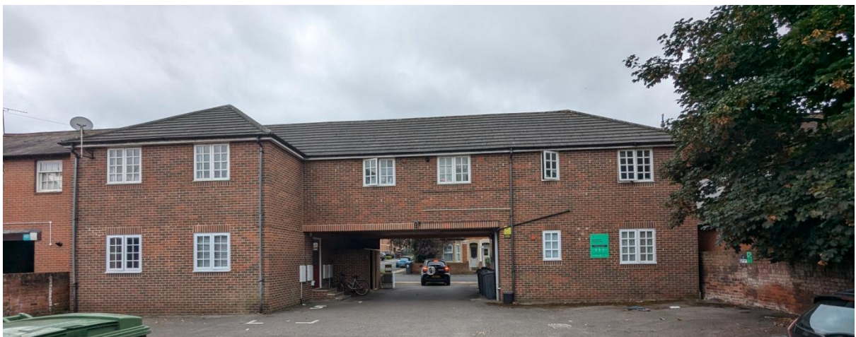
Rear view of 16 Goldsmid Road Block.
