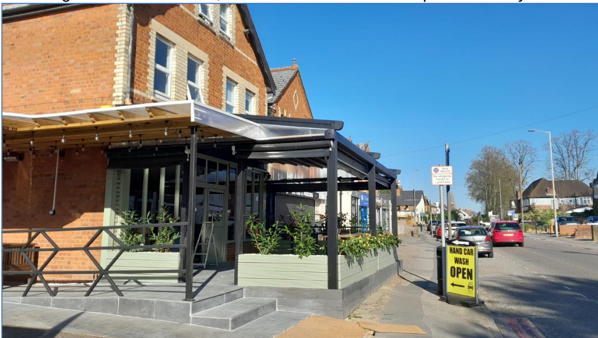
Fig 1. Front of 20 Norcot Road. Site photo taken by case officer on 20/04/2023
