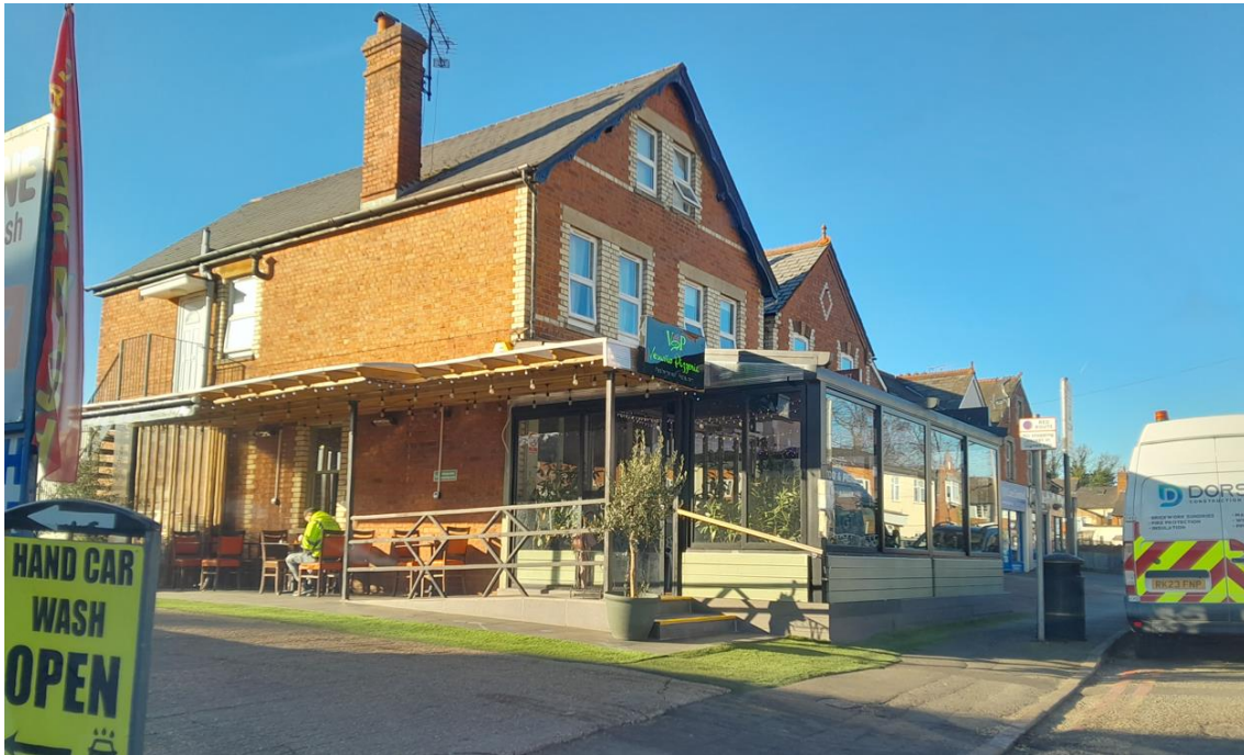
Fig 2. Front of 20 Norcot Road. Site photo taken by case officer on 16/04/2024
