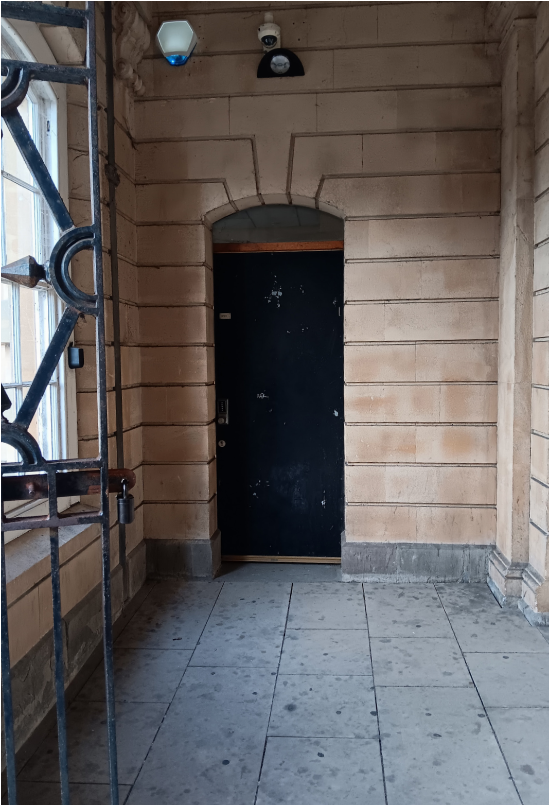
Fig.05 3. Existing door at restricted (north) entrance to be replaced..
