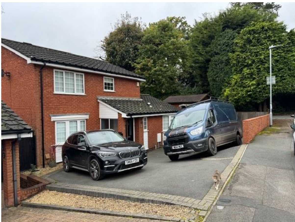
Site Visit Photos taken on 1 st of November 2024
