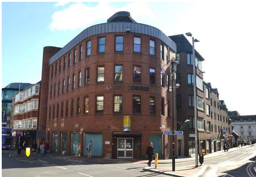
2-4 Kings Road situated on the prominent Abbey Corner- note the ground floor fenestration of little/no architectural merit
