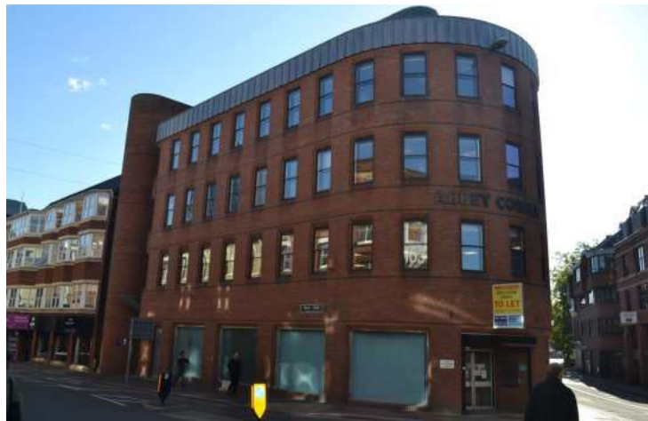
Ground floor of 2-4 Kings Road, Abbey Corner
