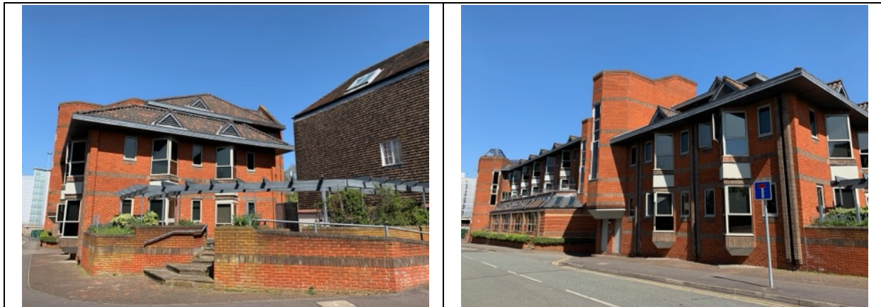
Figure 7 Milwards 1987 Headquarters and warehouse
