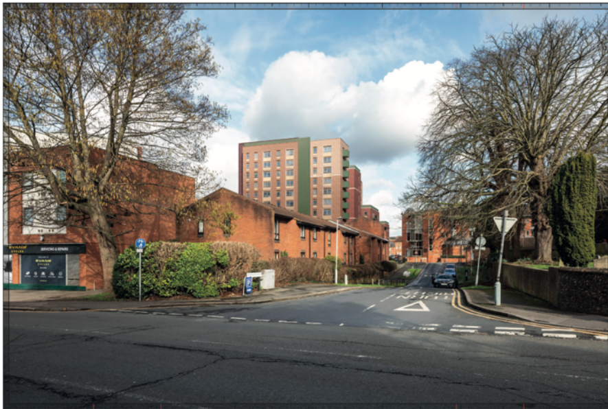
Figure 6 View east down Deansgate Road - cumulative
