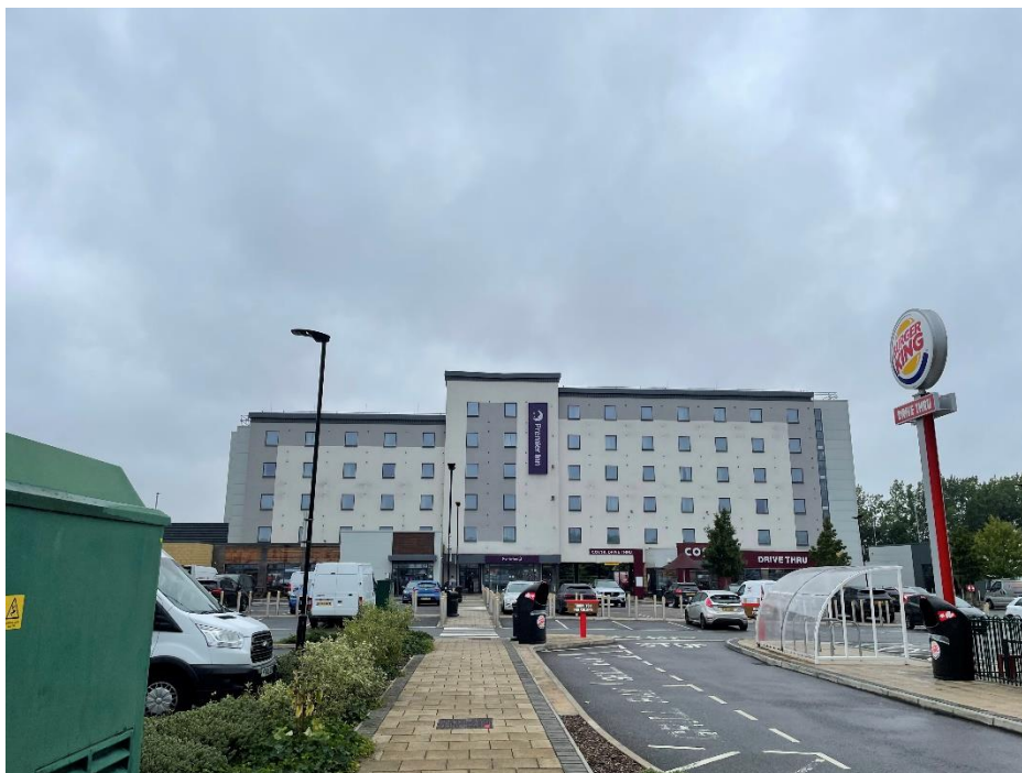
Reading South (Reading Gateway) Premier Inn (North Elevation)
