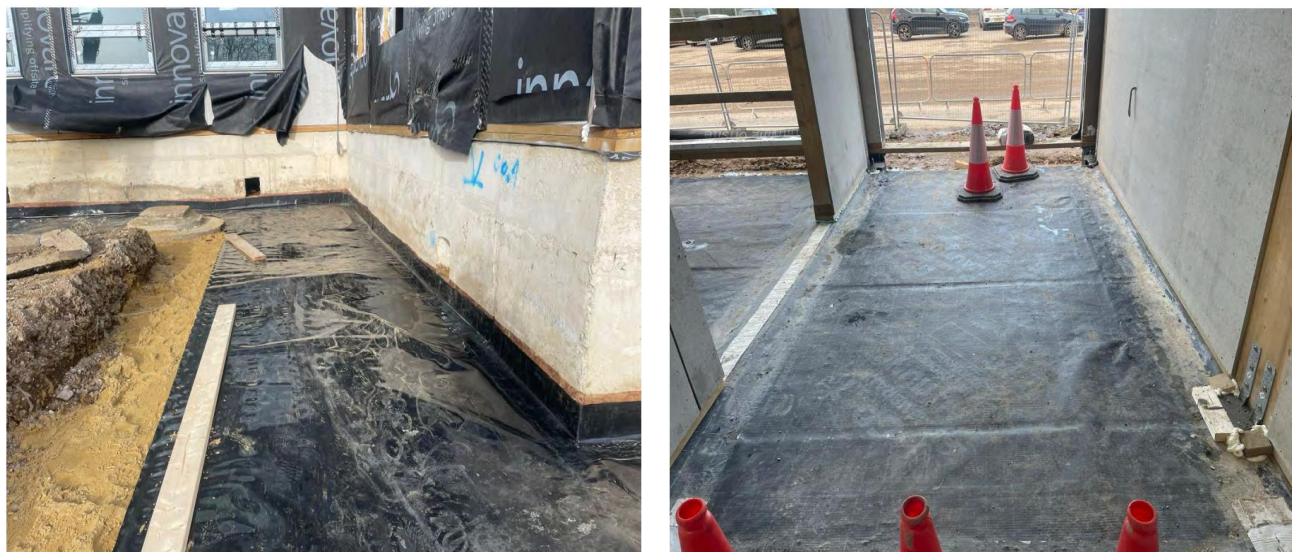
Figure 01 - Photographs of Geomembrane Cover
