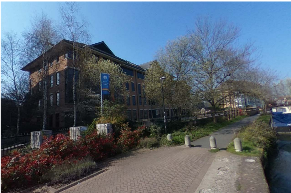
Figure 9 - View of Thames footpath looking West. The Thames footpath is illuminated with 4-metre tall functional LED floodlighting.
