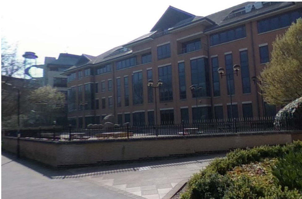
Figure 8 - View of rear terrace which uses the same 5-6 metre tall columns and decorative globe lanterns.
