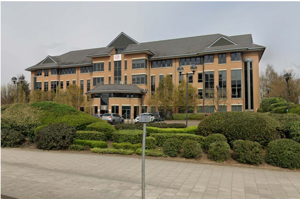
Figure 3 - View of front car park which uses 5-6 metre tall lighting columns with decorative globes.
