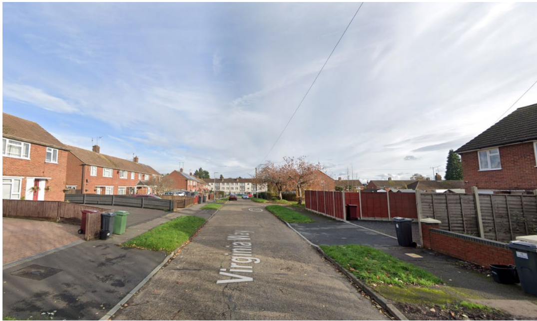
Fig 3. View east along Virginia Way, with the application site in the foreground to the right.
