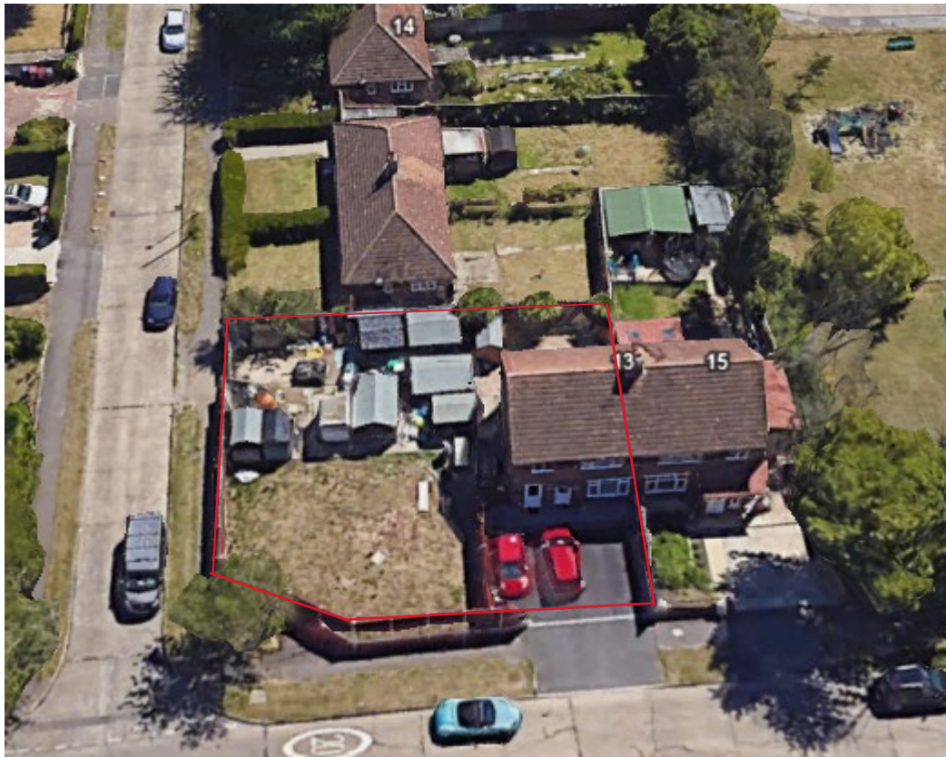
Fig 4. Raised view facing Maker Close and the site with the existing dwelling
