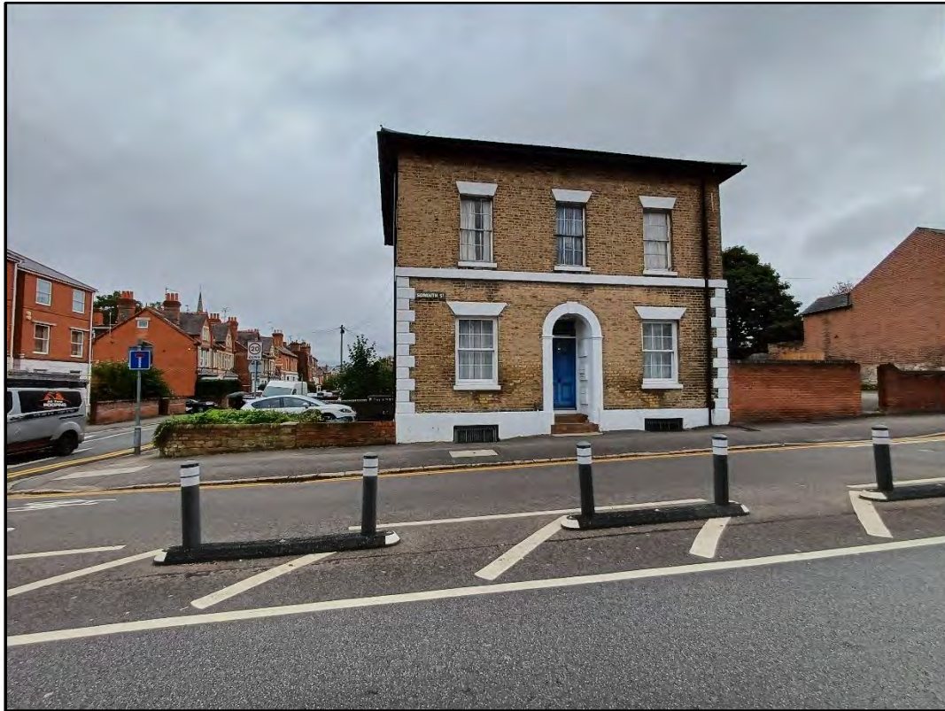
Plate 7: East-north-east facing view of 9 Sidmouth Street ( Asset 16 )
