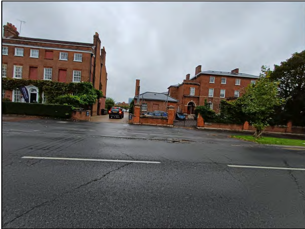
Plate 23: North-north-west view of Kendrick's View ( Asset 28 ) from London Road within Kendrick Road Conservation Area ( Asset 2 )
