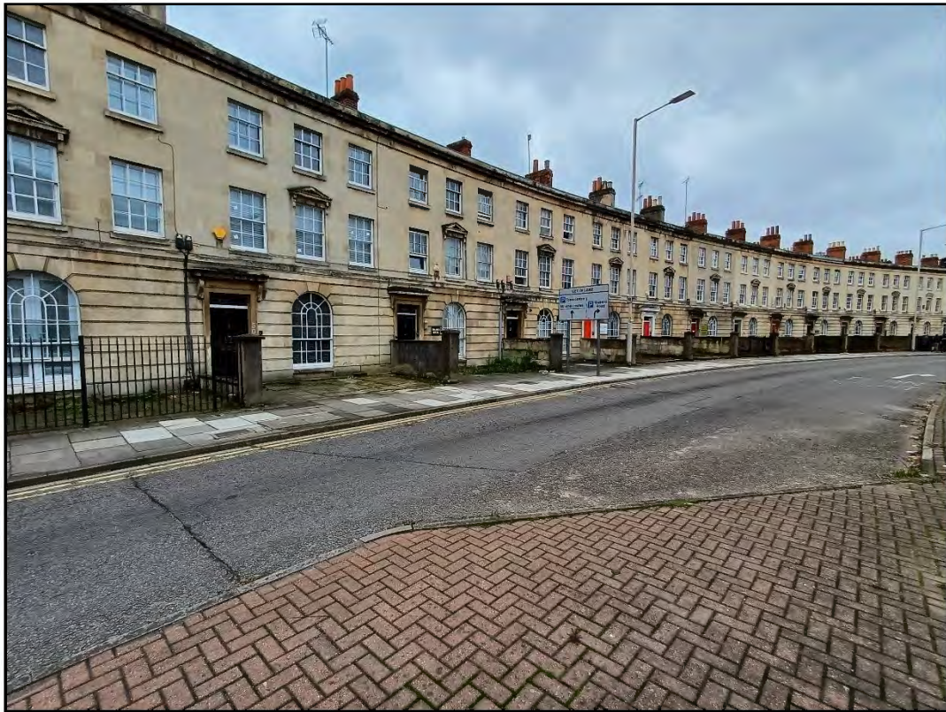
Plate 27: Southwest facing view of Queen's Crescent ( Asset 15 )
