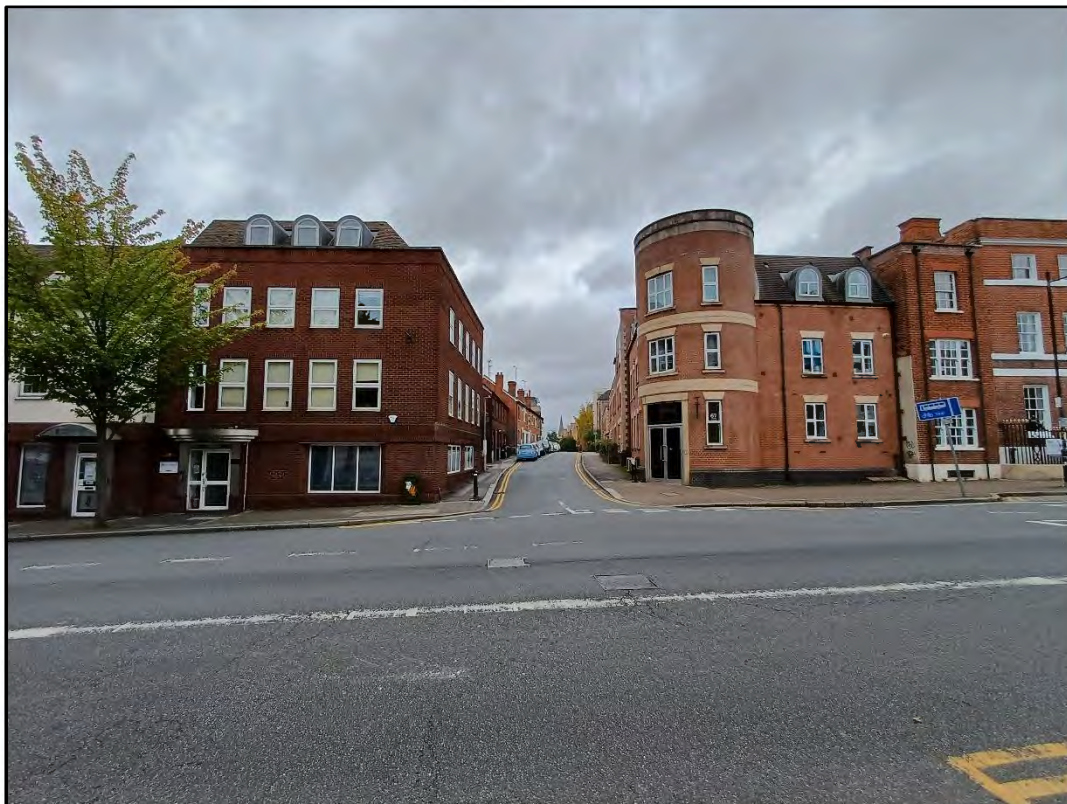
Plate 26: East-north-east facing view from London Street within Market Place and London Street Conservation Area ( Asset 3 )
