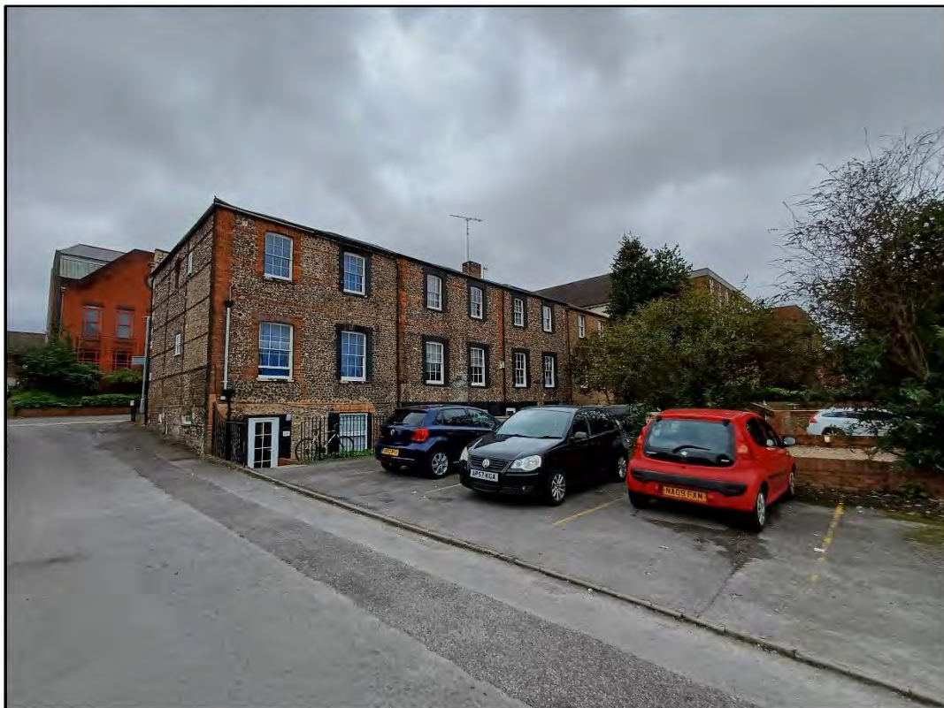
Plate 6: Southwest facing view of the rear of 43—49 South Street ( Asset 22 )
