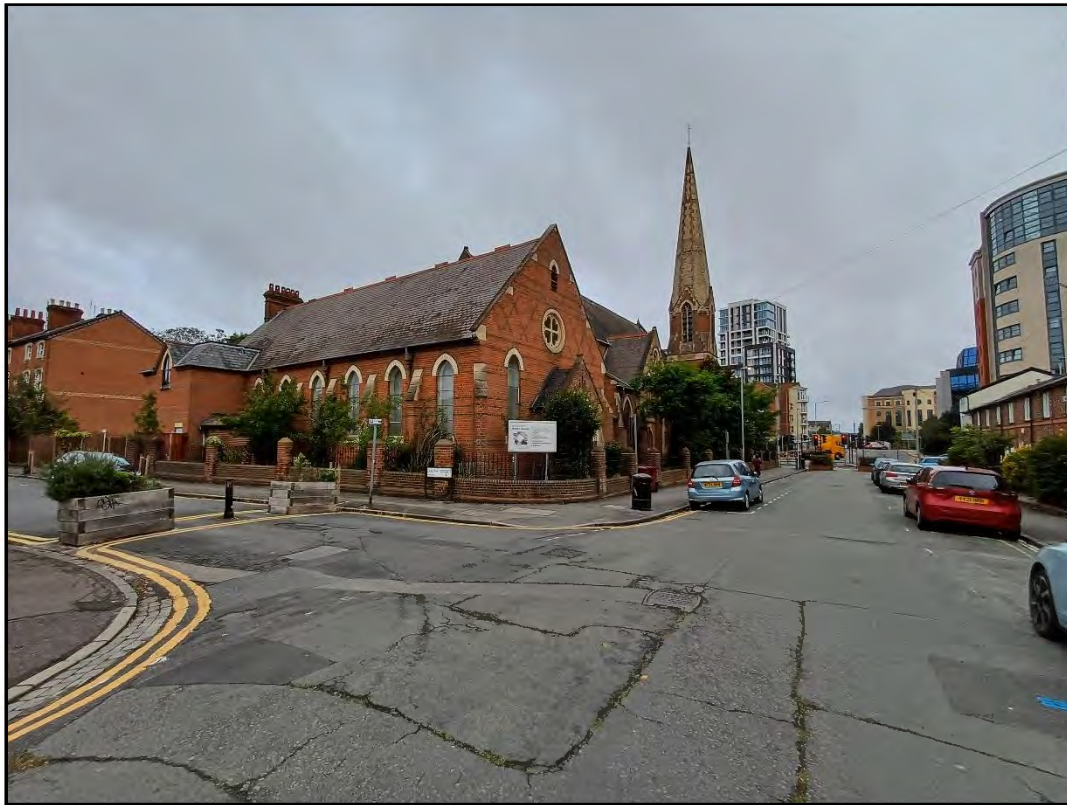
Plate 19: Northwest facing view of Wesley Methodist Church ( Asset 26 )
