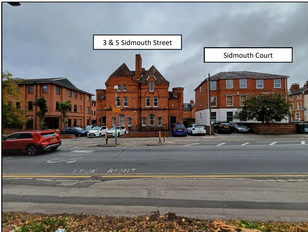
Plate 8: East-north-east facing view of 3 & 5 Sidmouth Street ( Asset 22 ) and Sidmouth Court ( Asset 87 )
