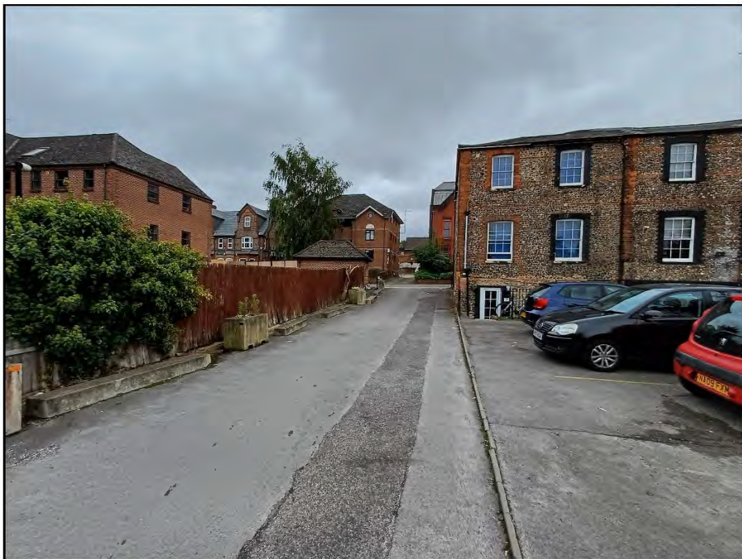
Plate 28: South-south-east facing view from outside Queen's Crescent ( Asset 15 )
