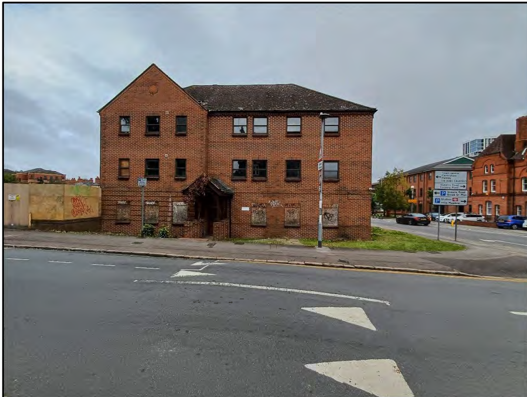
Plate 1: North-north-west facing view of Trinity Hall
