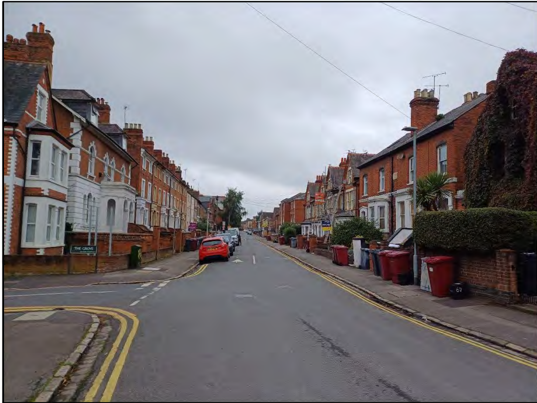
Plate 21: West-south-west facing from the westernmost edge of Eldon Square Conservation Area ( Asset 1 )
