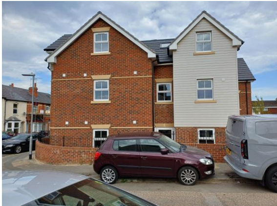
West side elevation of Block 1 building
