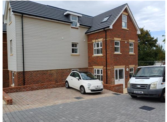
South rear elevation of Block 1 building
