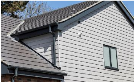
Light grey weatherboarding, with asphalt grey fascia boarding and painted window frames
