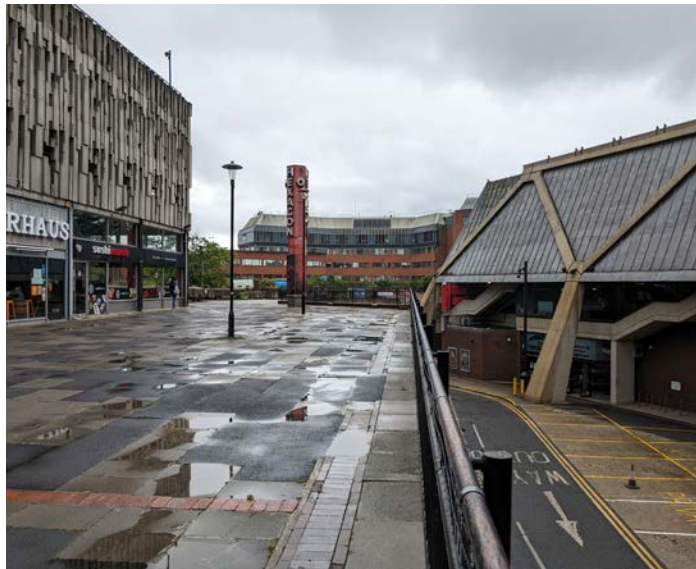
③ Existing surface materials and boundaries along Queens Walk
