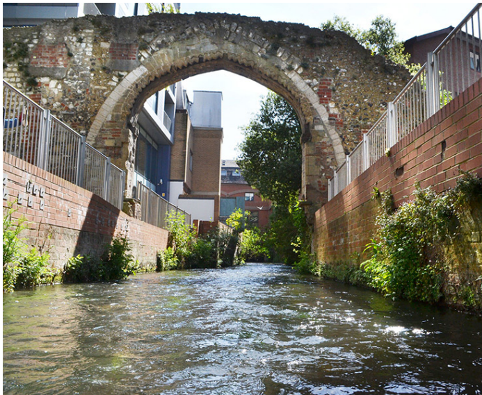
The Holy Brook beneath the old arch of the Abbey mill
