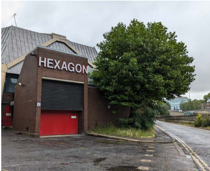
Existing London Plane (T1 in Tree Survey) on the west side of the Hexagon, regularly pollarded
